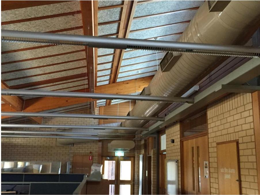
Ceiling in the 1981 addition, note the use of similar materials to the 1975 section, however, the quality of the detailing is not as high and the bespoke light fittings, which are a feature of the building are not included.
