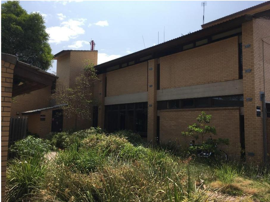
View of northern elevation showing the addition of the lift tower, off-form concrete as a decorative structural element and cream face brick.
