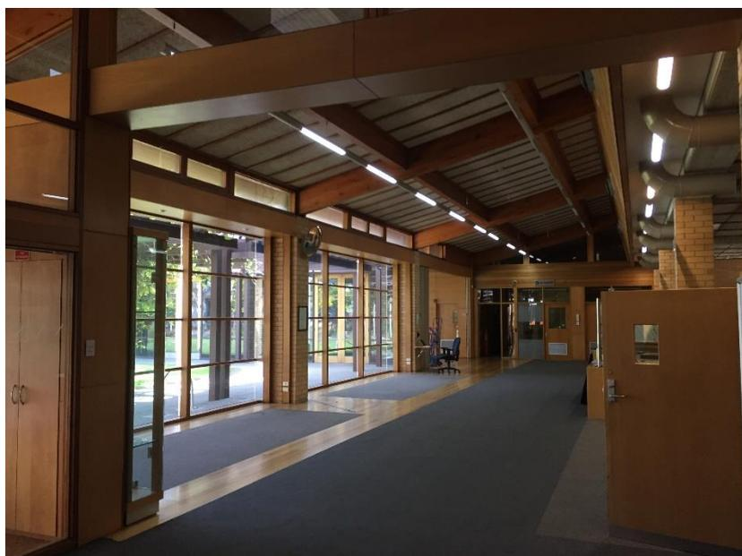
View of the front of the 1975 building, this space was once the Exhibition Hall, the wall has been slightly pushed out and replaced with glass. Note the difference in the framing between the original windows above.
