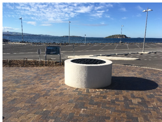
Site works complete June 2019 Source DEW
