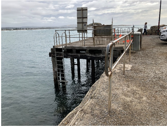
Rosetta Head Jetty 4 March 2020 Source DEW
