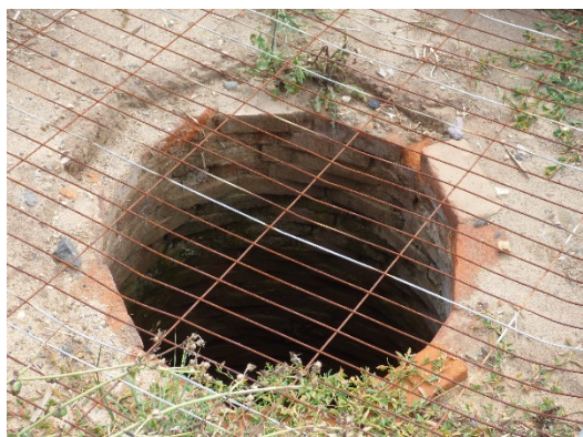
Uncovered well 23 November 2017 Source DEW
