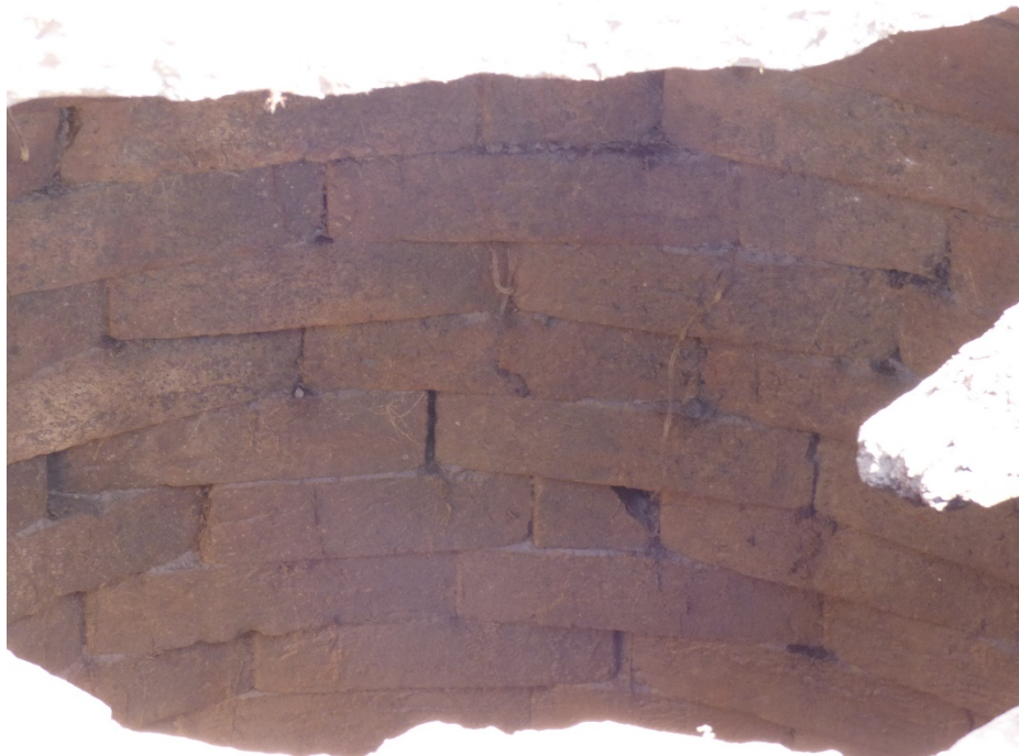
Close-up of brick lining of the well 17 March 2017 Source DEW
