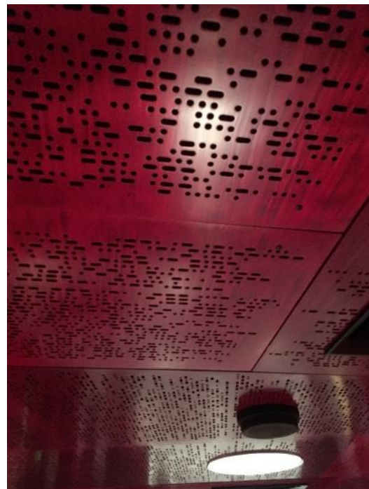
Timber panel ceiling in the theatre, the dots and dashes are words depicted in Morse code.
