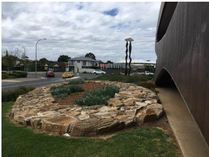
'O' formed from roughhewn rocks, cemented in place.
