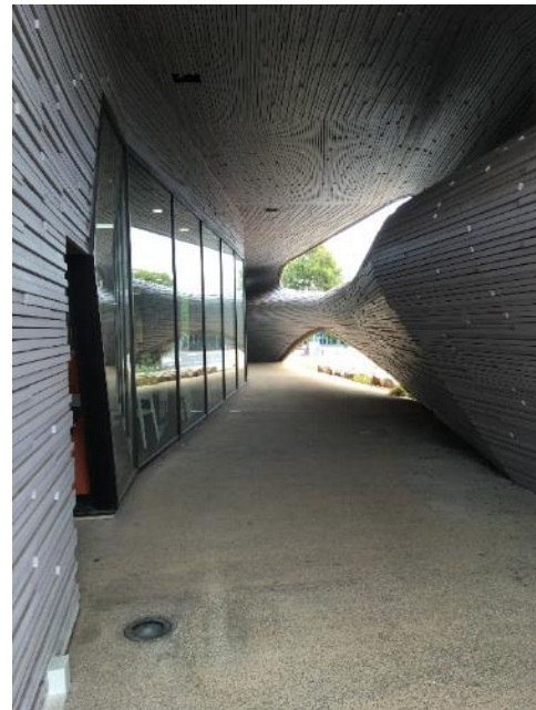
Passageway created down the side of the building by the extruded R. Note the painted timber batons.
