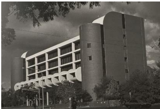
Fire Services Headquarters, SHP 26356
