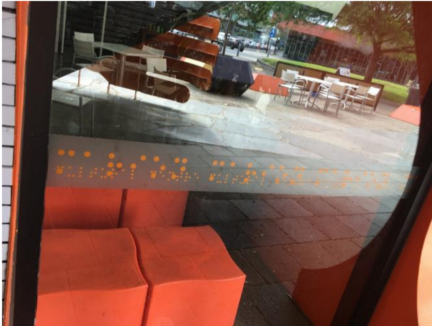
Braille panel extending along the glazing. The large dots denote 'marion', the small dots underneath denote 'cultural centre'.
