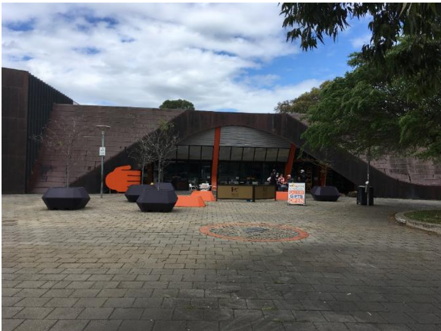
North-western façade showing the courtyard facing the café.
