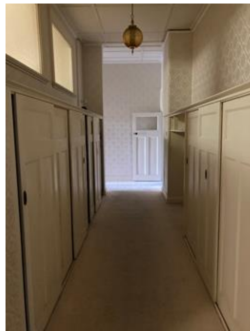
View of internal corridor showing original cupboards and ceiling
