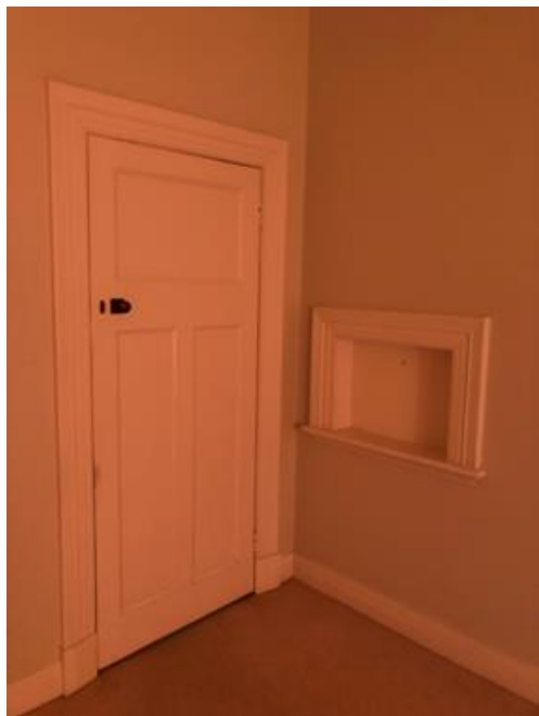
Origin door and hatch to kitchen in the dining room
