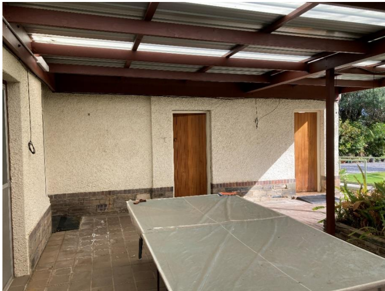
View of covered external courtyard, formed between the two wings of the house
