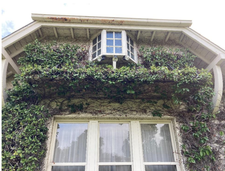
Detail of front gable note the 'dormer' window, cantilevered concrete hood, decorative timber framing, and probably the replacement of the 'lead-light' multi-pane windows in the upper half of the window with a single pane of clear glass
