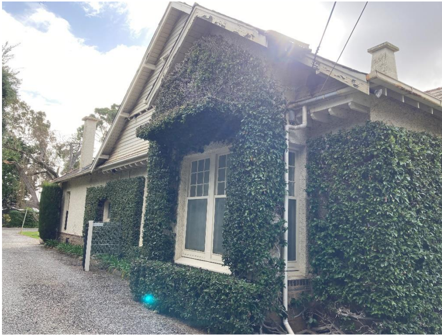
View of western elevation, showing bay window and example of the cantilevered concrete window hoods
