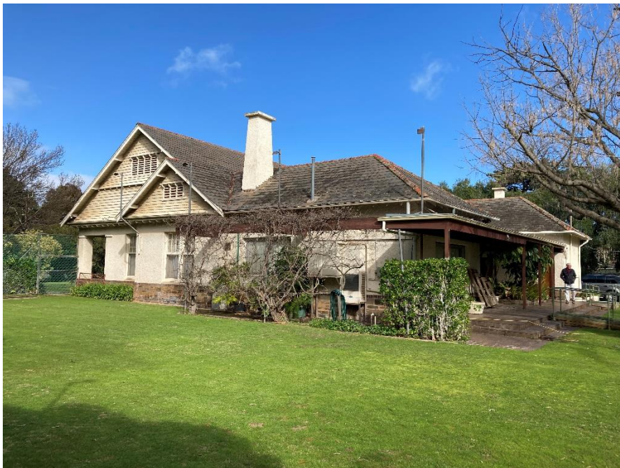
View of eastern elevation, note the scallop detailing and vents in gable ends
