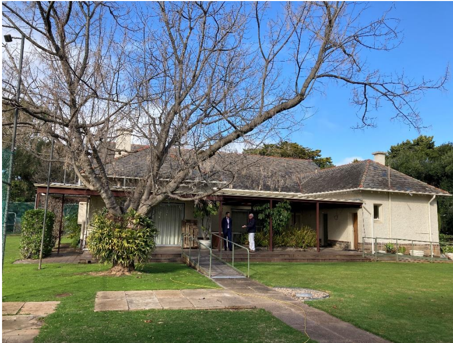
View of southern elevation, note the enclosed courtyard between the two rear wings to the right are the laundry and external toilet, on the left is the kitchen and sunroom with large glass sliding doors
