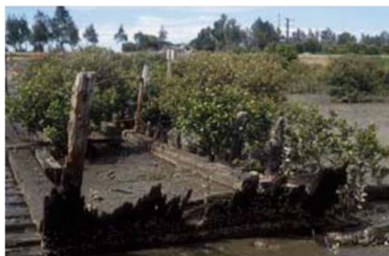
The remains of the Fish Market Pontoon at Jervois Basin
