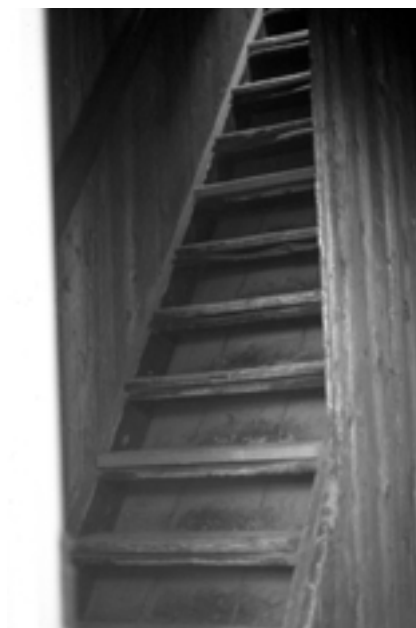
Figure 44 Stair, Portable Iron Houses, South Melbourne, VIC.
