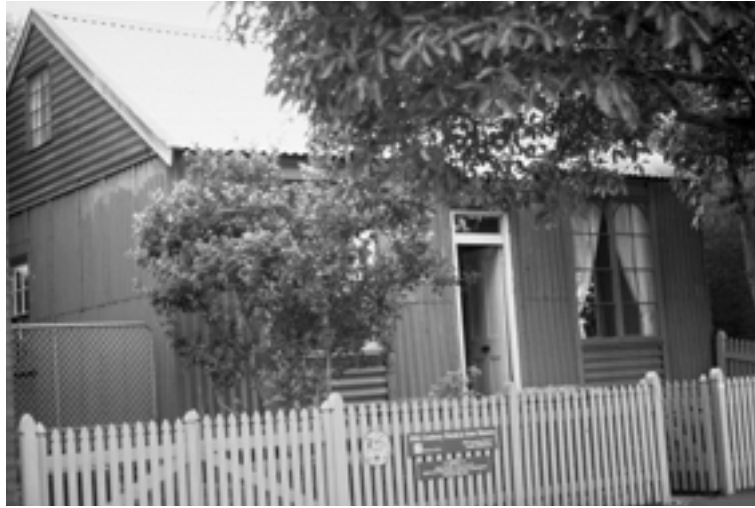
Figure 43 Portable Iron Houses, South Melbourne, VIC. The small attic rooms are accessed by a steep narrow stair.
