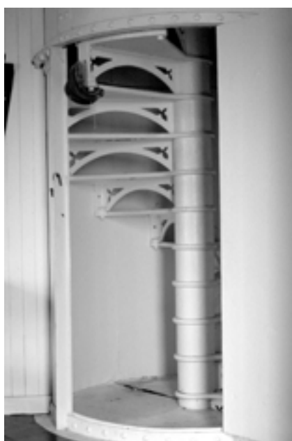
Figure 42 Cape Jaffa Lighthouse, Kingston, SA. Narrow curved stairs are the only means of access to the upper levels.
