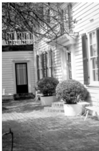
Figure 10 Mulberry Hill, Baxter, VIC. The existing parking space is some distance from the building, but a designated space is to be located near the principal entrance.
