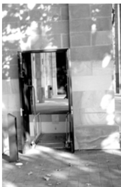
Figure 22 Platform Lift at the Courts Building, Angas Street, Adelaide, SA. Unfortunately this requires attendants to operate it, which means it is not independently accessible.
