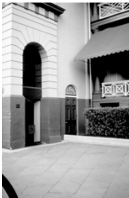
Figure 21 Parliament House, Sydney, NSW. A former window has been extended to ground level to provide access to a lift, thereby overcoming the problem of the adjacent 13 steps.
