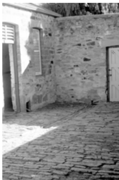
Figure 14 Police Stables, Burra, SA. The rough cobblestones are difficult for anyone to walk over. One solution to this situation is a new timber boardwalk above the cobblestones to guide patrons to each item of significance on display.
