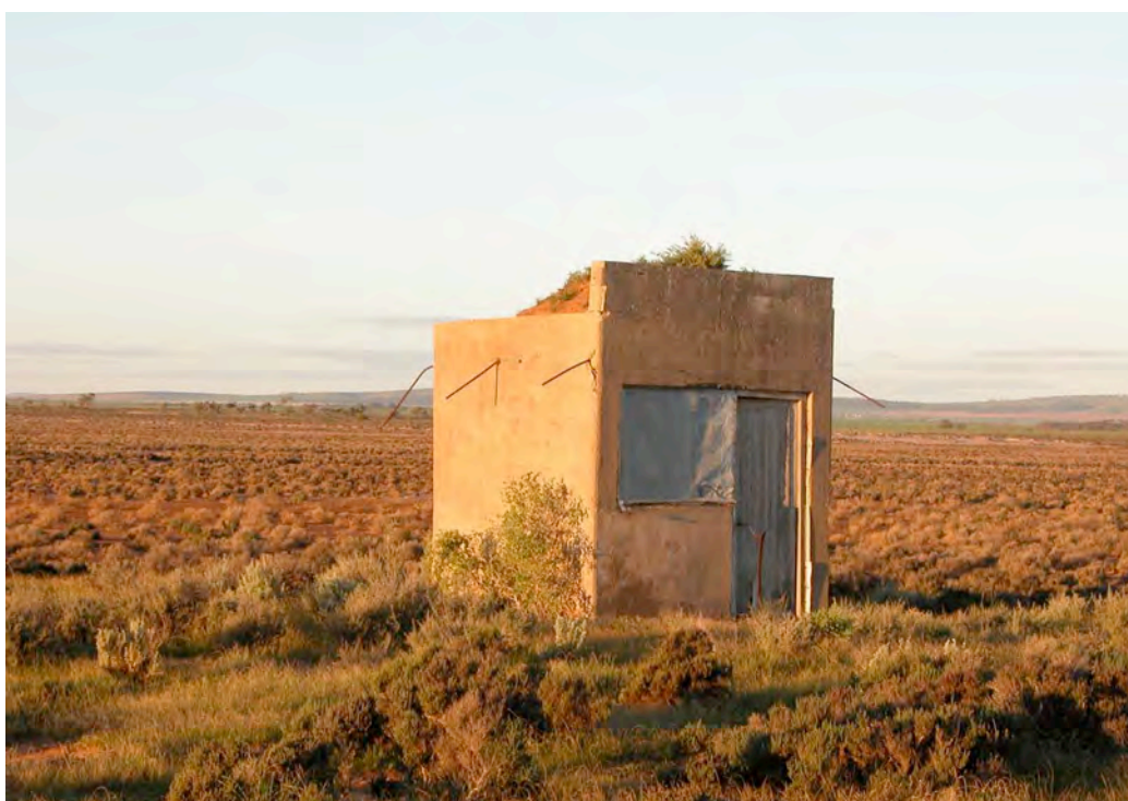
One of two concrete shelters at Gunnery Range
