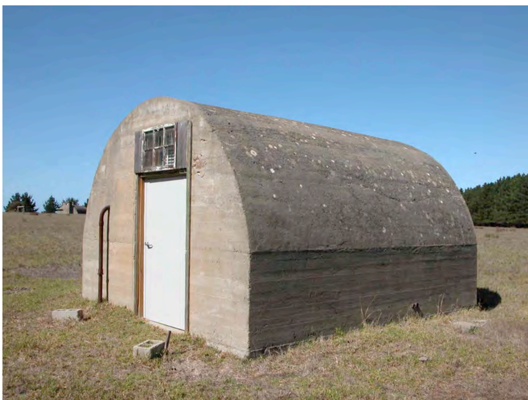
Generator building, Victor Harbor Radar Station
