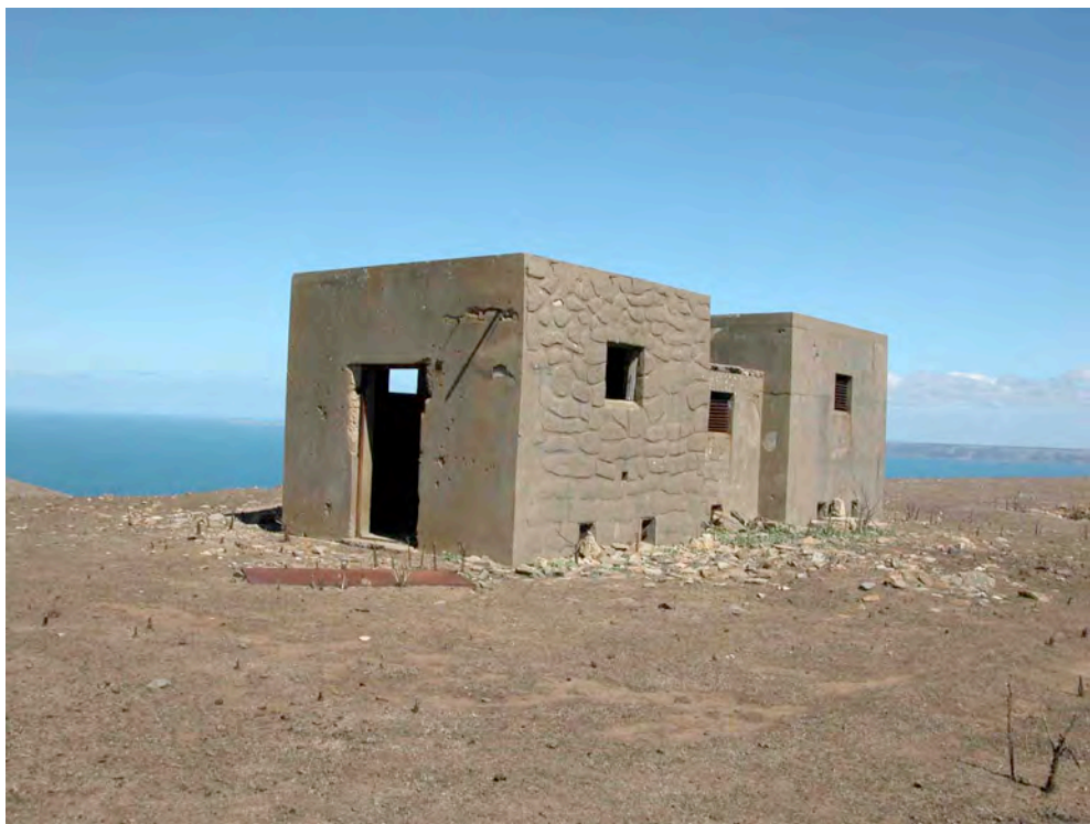
Transmitter & receiver building, Cape Jervis Radar Station
