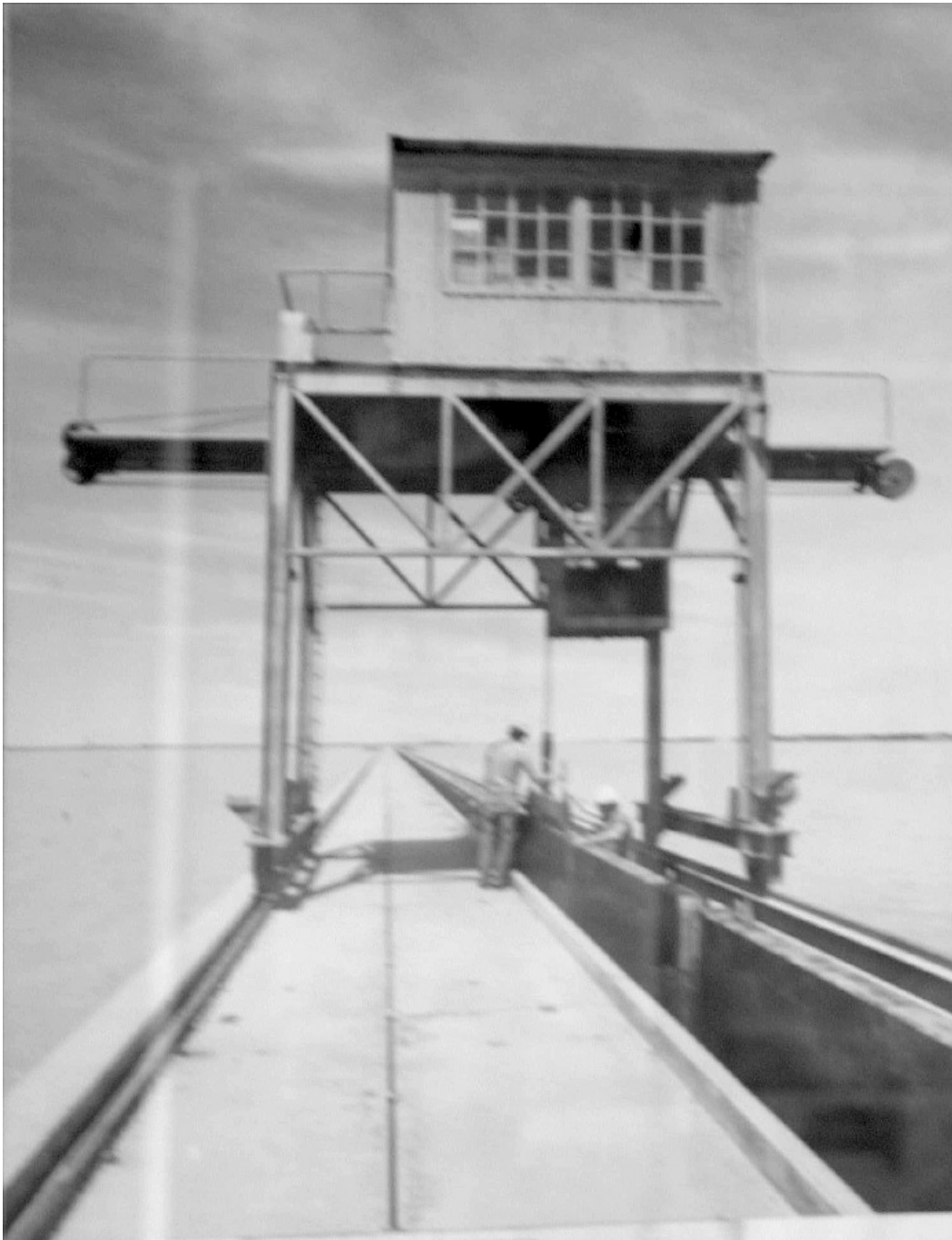
One of the travelling gantries opening a sluice gate on the Tauwitchere Barrage. The gantries were scrapped about 1990, and replaced by truck-mounted cranes. (E&WS interpretation sign, Goolwa)
