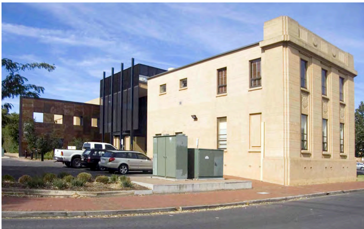
City of Mitcham Council Chambers, looking south-west
