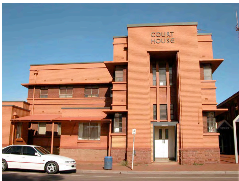
Whyalla Court House from north-east
