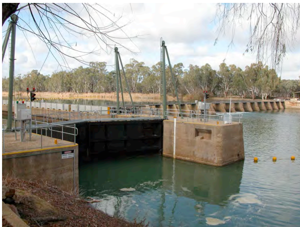
Lock 2 at Taylorville near Waikerie, built 1928
