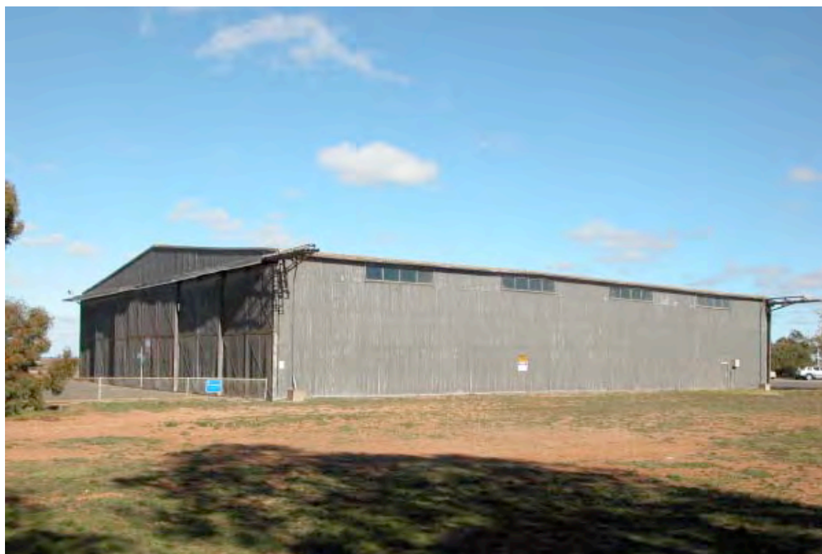
Bellman Hangar remaining at RAAF Port Pirie
