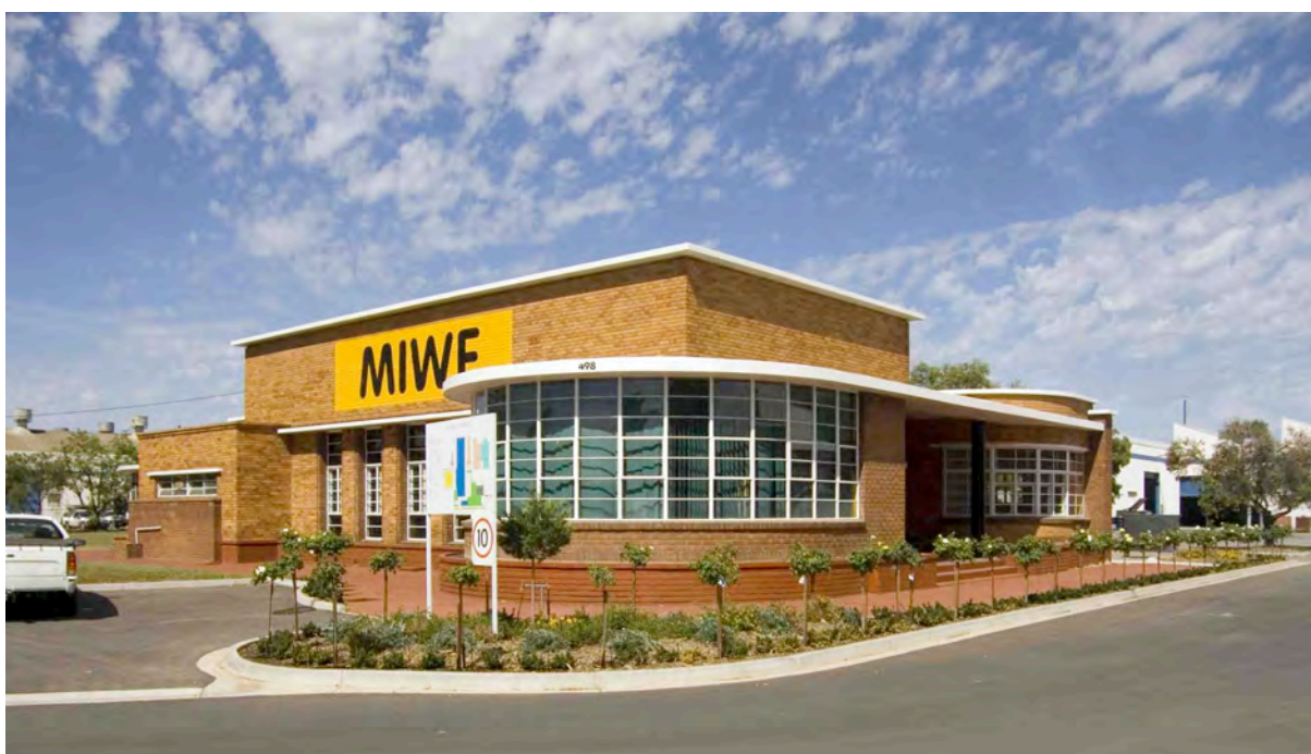
Former Tubemakers Administration Building 2, looking south-west
