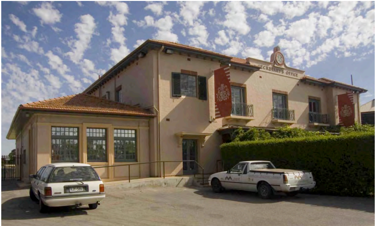
Adelaide Showground buildings, Secretary's Office looking south-west
