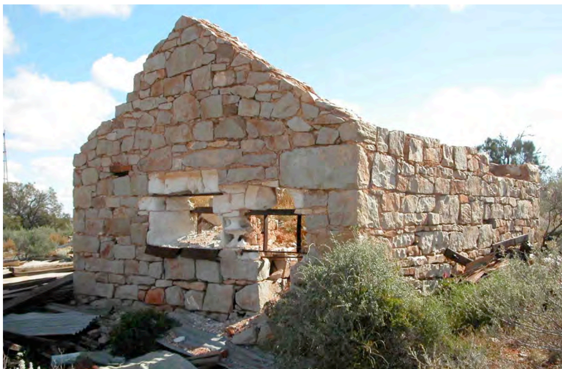
Tarcoola bakery (?) ruin, looking north-west
