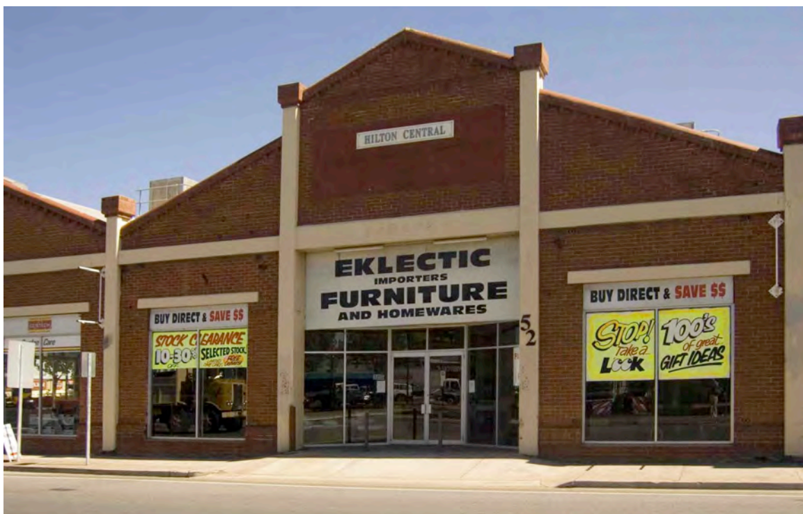
Former AESCO Limited buildings, 1924, looking north
