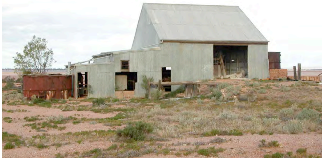
Glenloth Battery, looking south-east, Lake Harris in background
