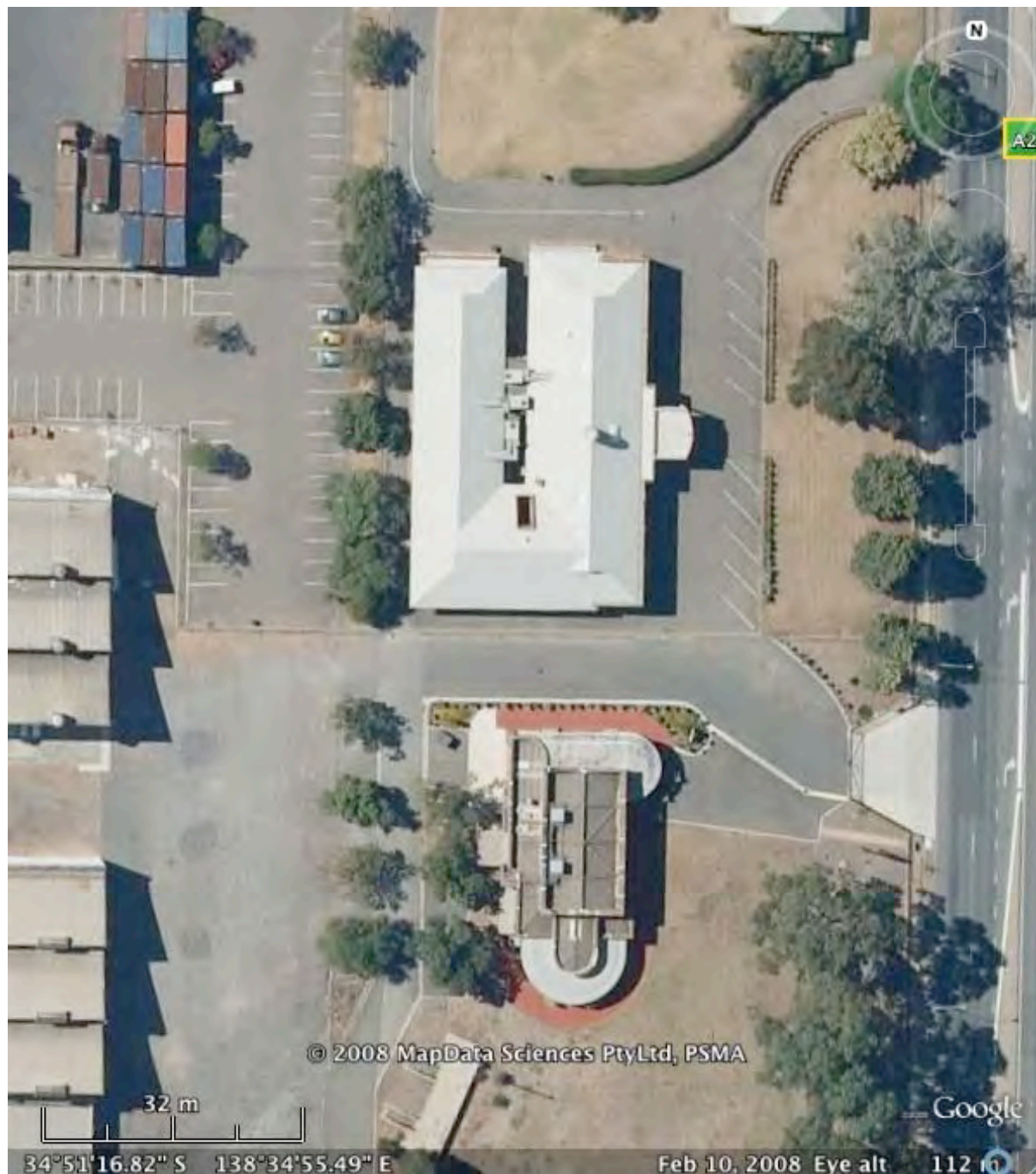
Aerial view of Former Tubemakers Administration Buildings 1 and 2
