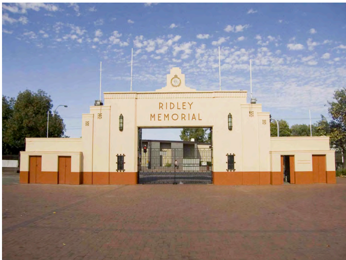
Adelaide Showground buildings, Ridley Memorial Gates looking west
