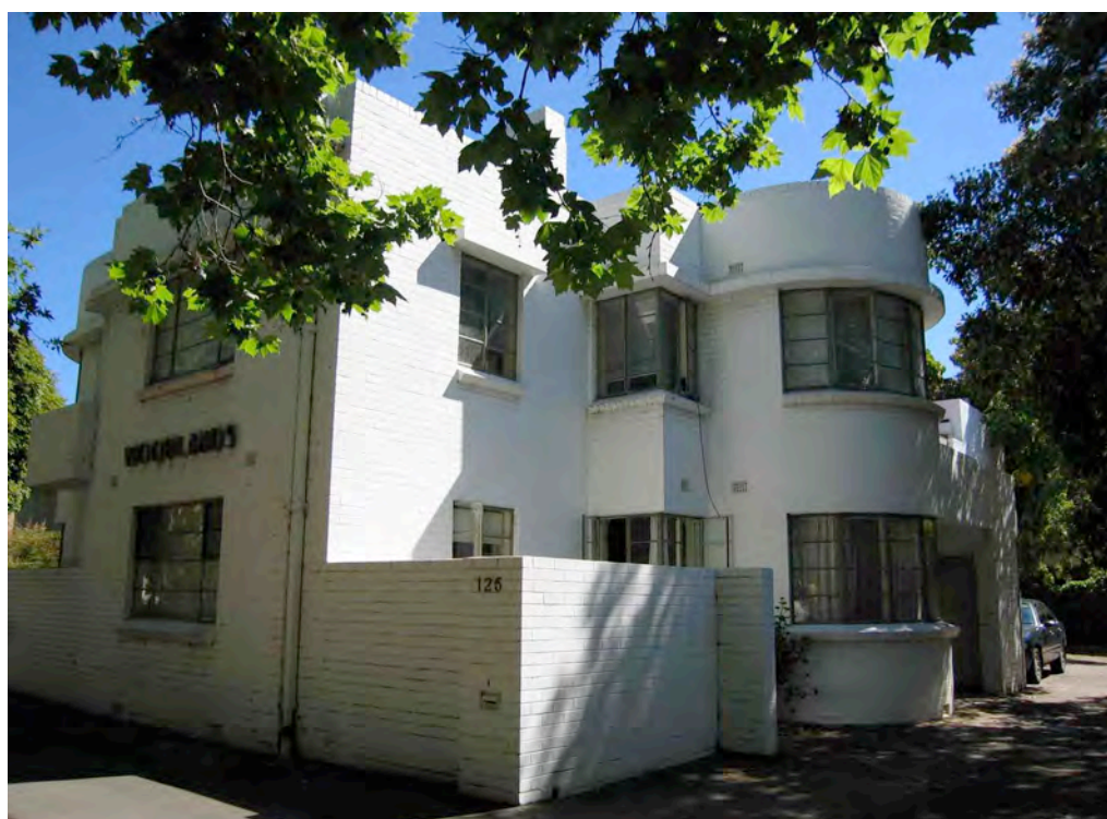
Woodlands apartments, looking south-west
