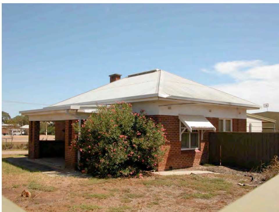
Caretaker's Residence, Parafield Airport (1929)
