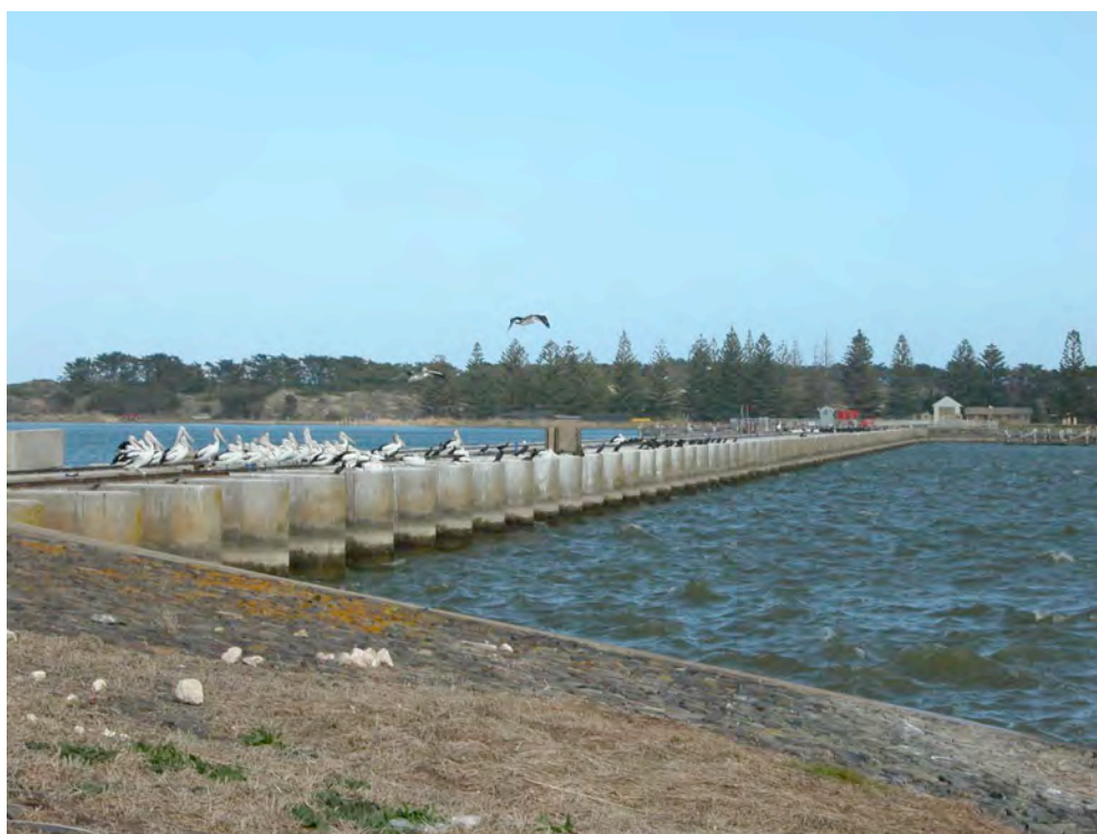
Goolwa Barrage, looking south
