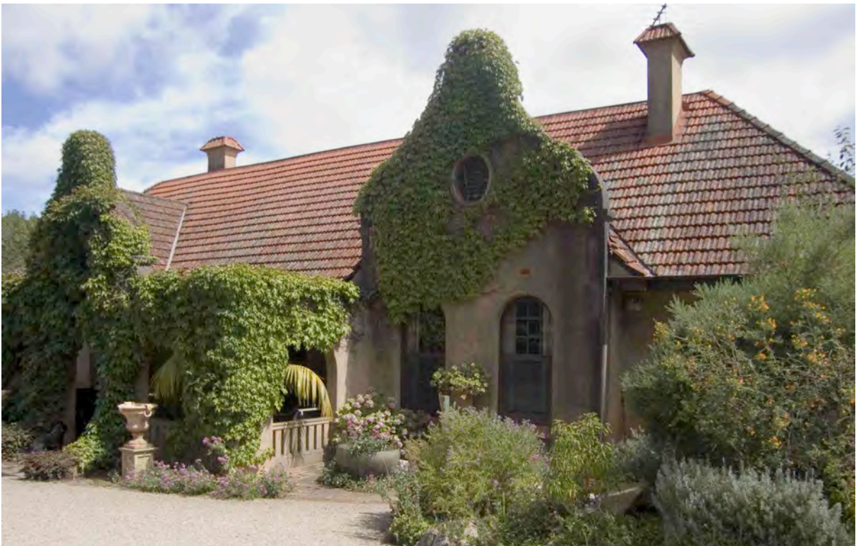
Scammell residence, Beaumont, looking north-west
