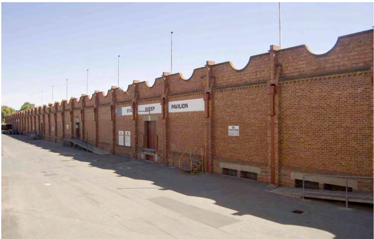
Adelaide Showground buildings, Wool Pavilion looking south-west
