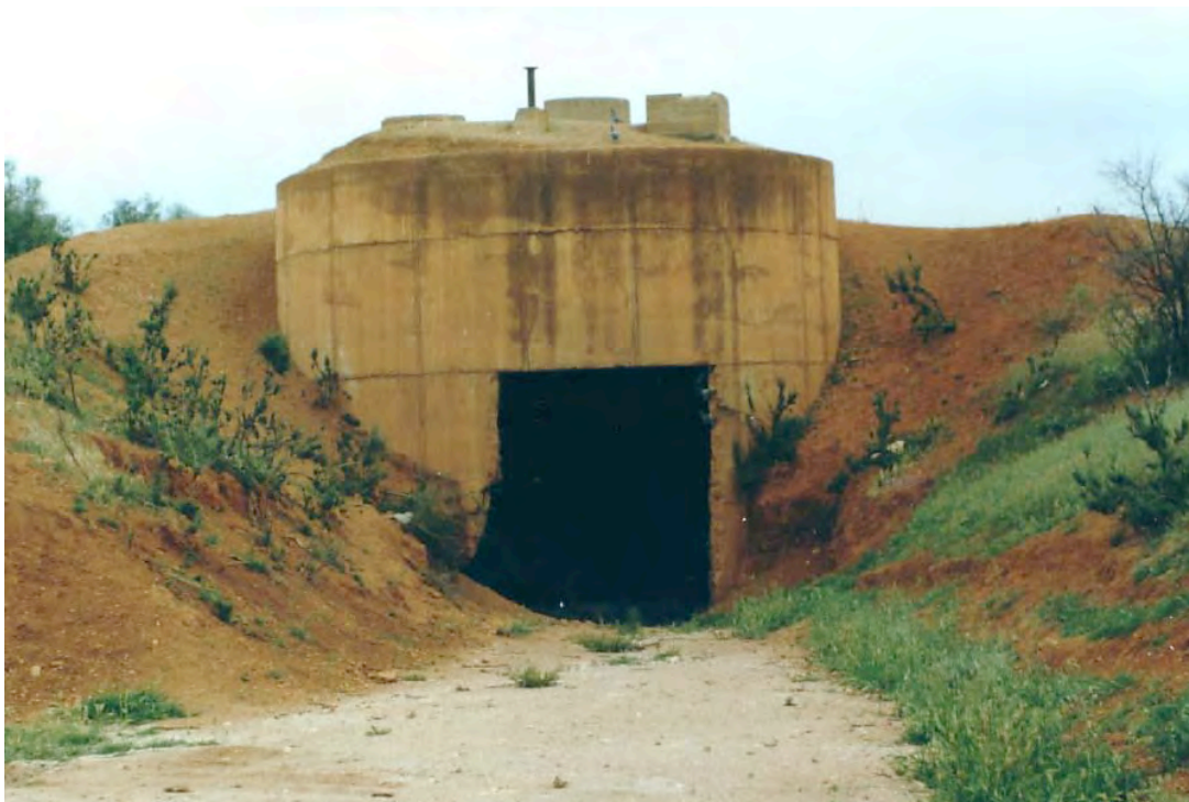
28 IAFD Gladstone, fuel tank cut open to remove steel lining
