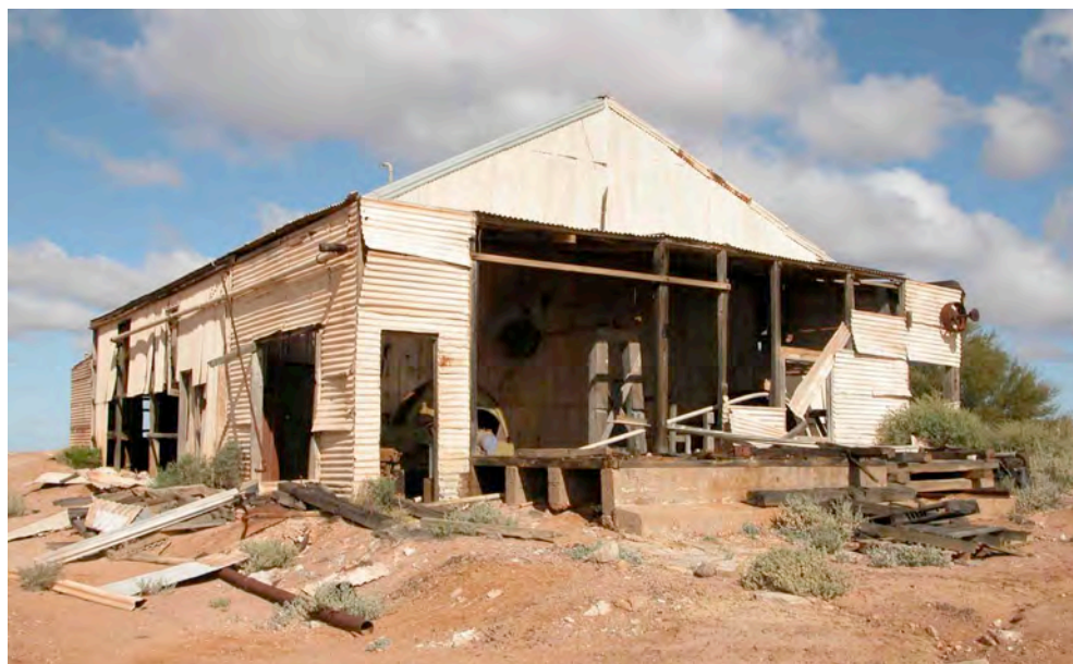
Tarcoola Battery, looking south-west, showing recent storm damage
