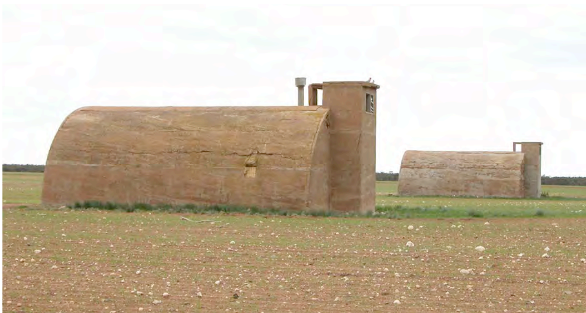
Transmitting and receiving shelters, Cowell Radar Station
