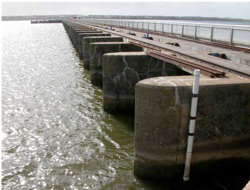
Goolwa Barrage, looking north
