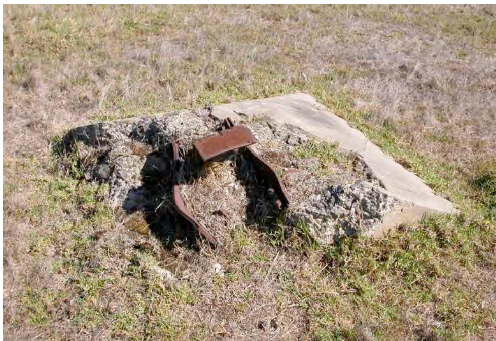
Footing of demolished timber tower at Radar Station
