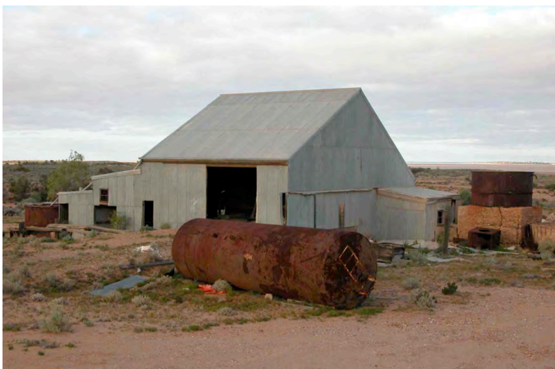
Glenloth Battery, looking north-east, abandoned boiler in foreground
