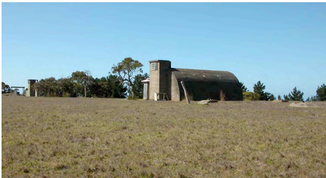
Radar transmitter and receiver buildings, tower base at right
