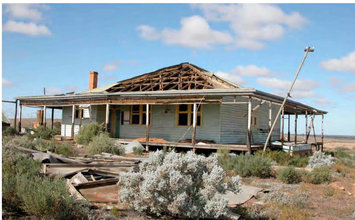
Tarcoola Homestead, looking south-east, showing recent storm damage
