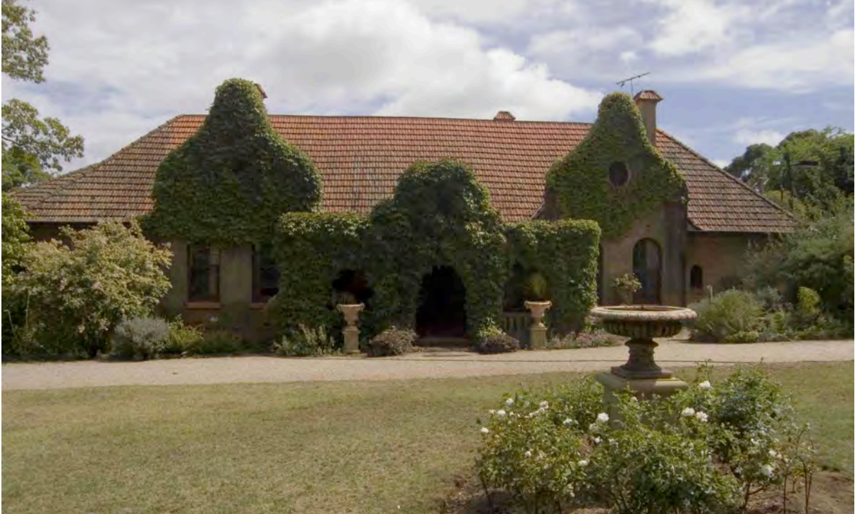
Scammell residence, Beaumont, looking north
