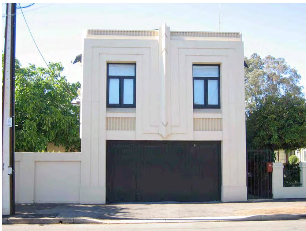
3A Prospect Road, looking north
