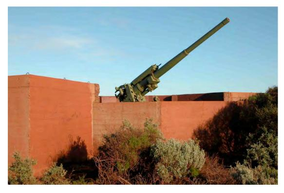
Anti-Aircraft Gun Emplacement fitted with a 3.7 inch gun
