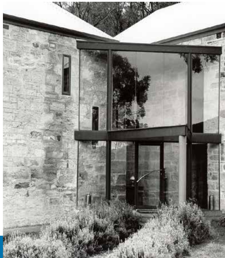
New Glass and steel entry lobby to the former Balhannah Mine, now converted to a dwelling
