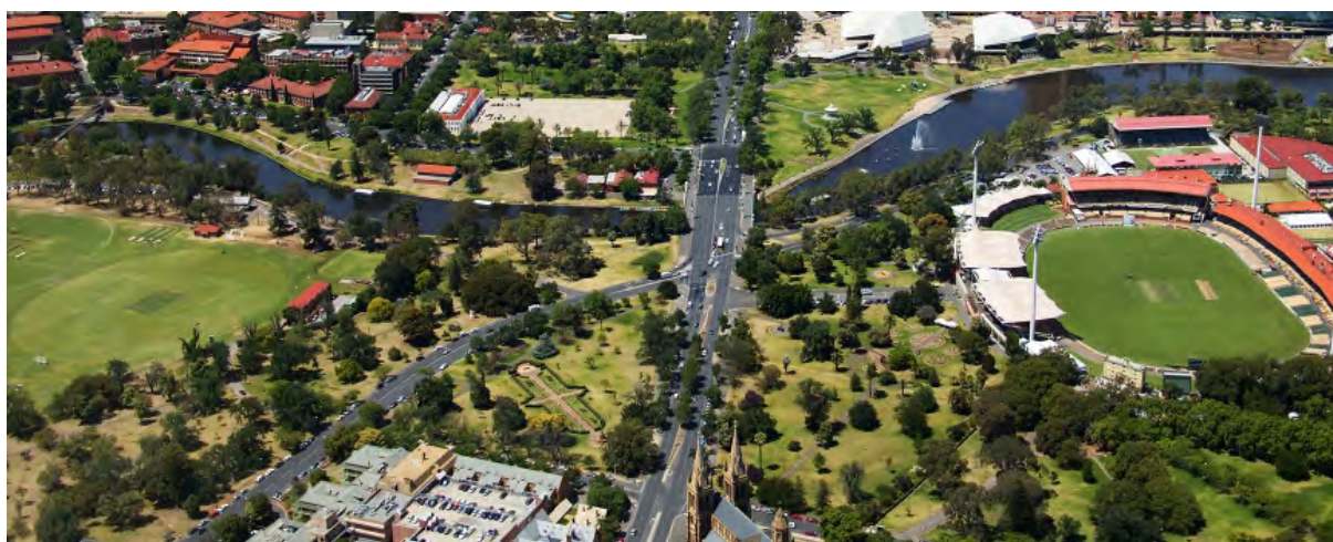
Figure 33 – Aerial view of Adelaide Oval and Torrens
