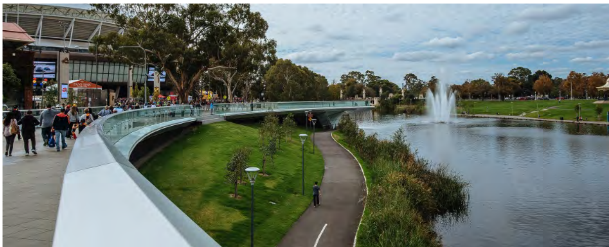
Figure 35 – Adelaide Oval footbridge over the Torrens (Park 26)
