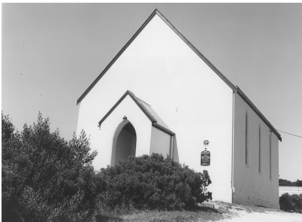
Former Robe Bible Christian Chapel prior to restoration, c1983, showing flush-rendered walls.
