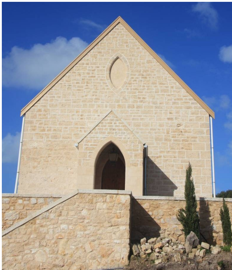
Former Robe Bible Christian Chapel, 6 August 2013, showing north elevation with porch and reinstated blind gable opening.
