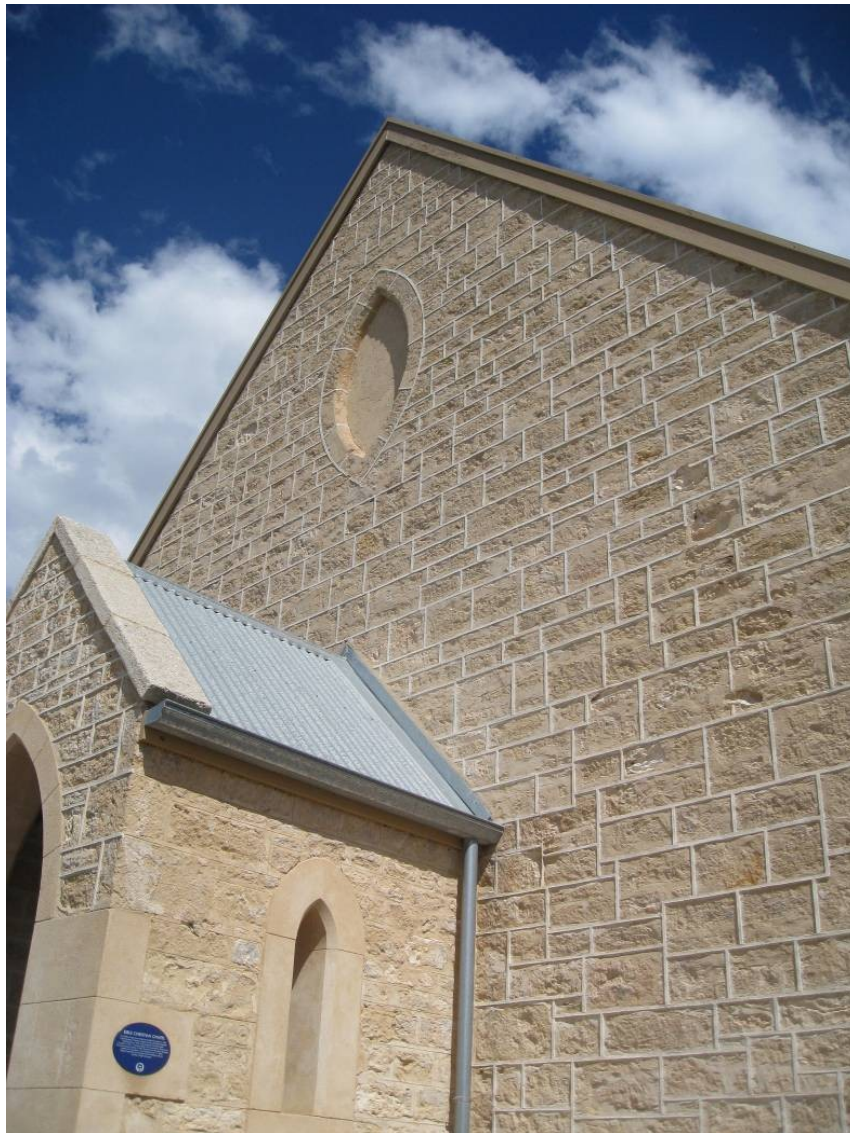
Former Robe Bible Christian Chapel, 9 February 2021, restored façade and porch showing tuck pointing.
