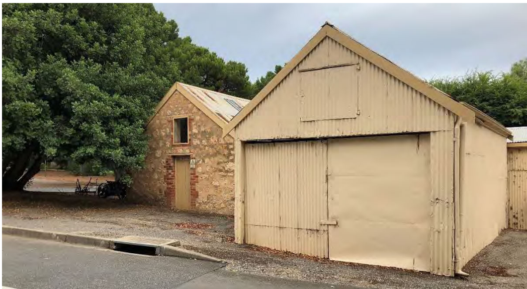
Figure 12: outbuilding with lightweight addition to older masonry section (GGA, February 2021)
