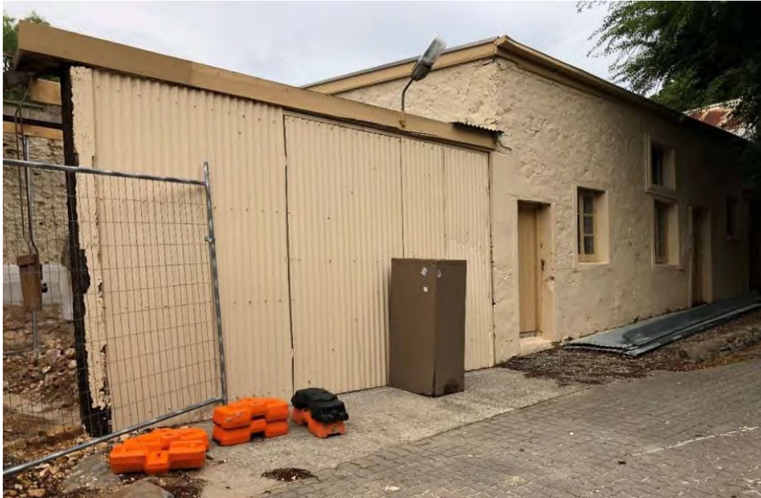
Figure 13: outbuilding with lightweight addition to older masonry section; collapsed wall at left (GGA, February 2021)
