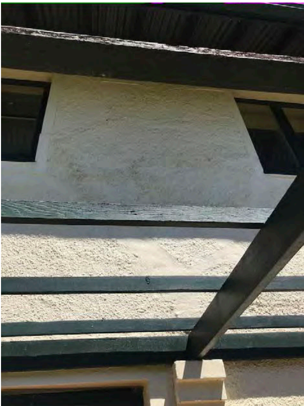
Figure 19: Previous repairs and cracking to masonry walls of double-storey wing Source: Hosking Willis, 2020
