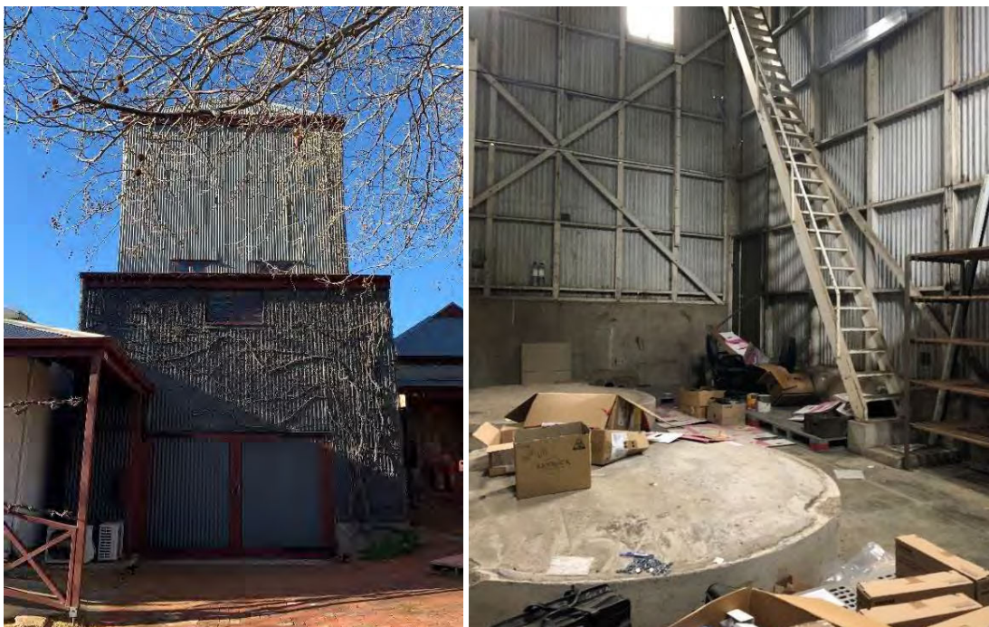
Figure 17, 18: Exterior of Still House, and internal view showing concrete bases for stills (GGA, February 2021)
