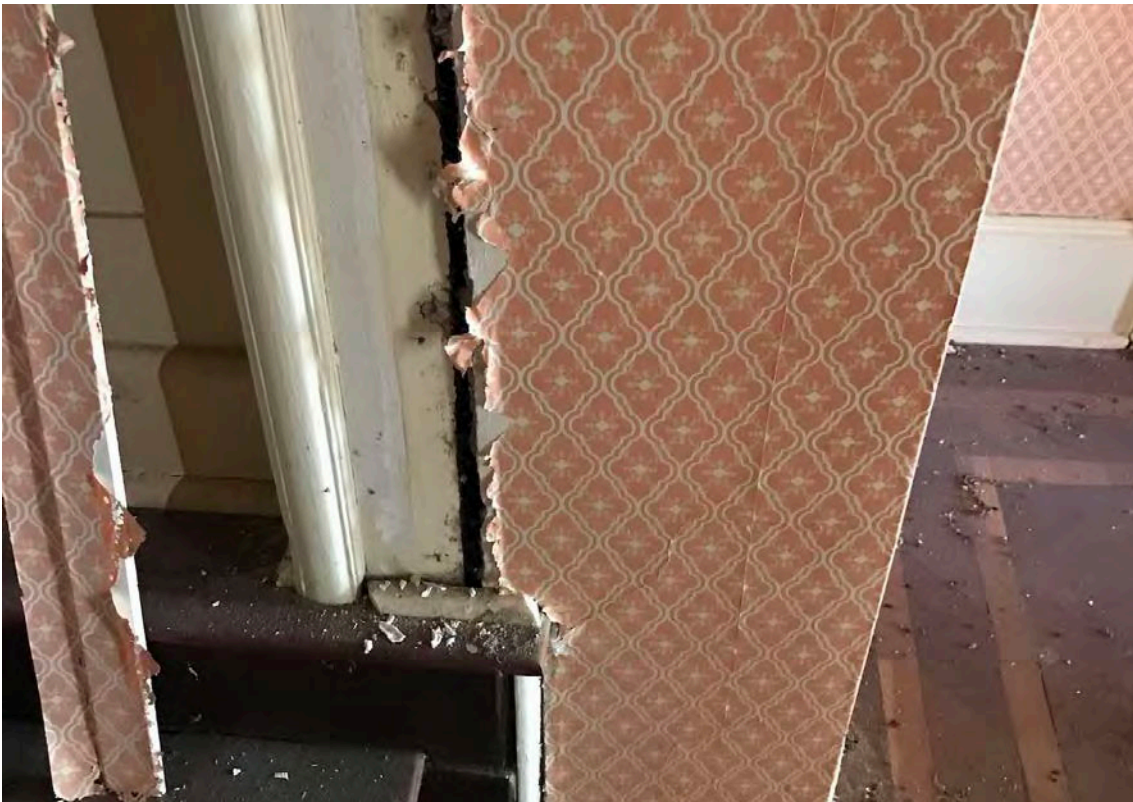
Figure 14: Internal junction of timber dwelling (left) and brick two storey wing (right)
