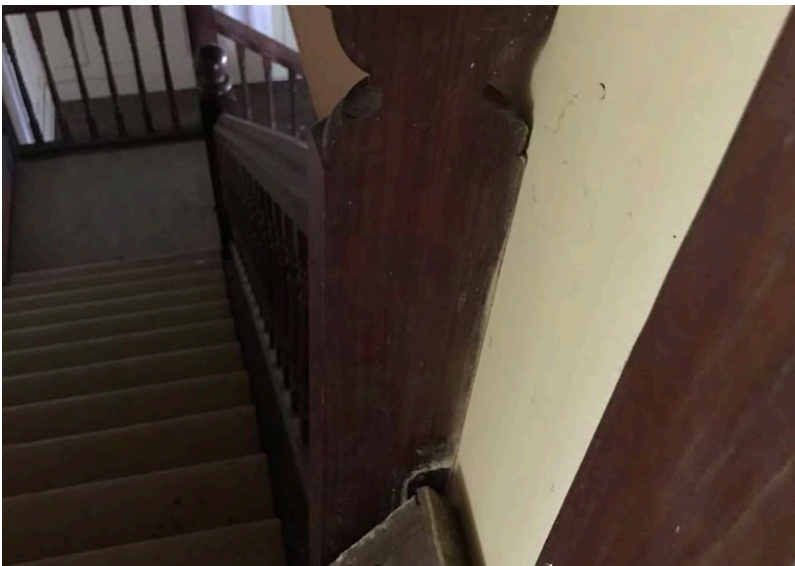
Figure 16: Incongruous fitting of internal stair with half newel post Source: Hosking Willis, 2020
