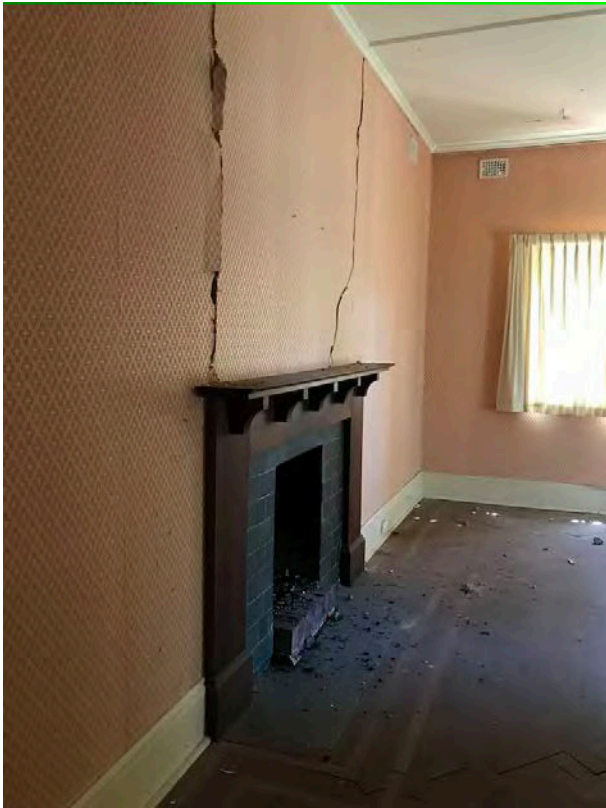
Figure 20: Cracking and damp to masonry walls of double-storey wing. Significant settlement along eastern side of the wing has resulted in major bowing of floor structure
