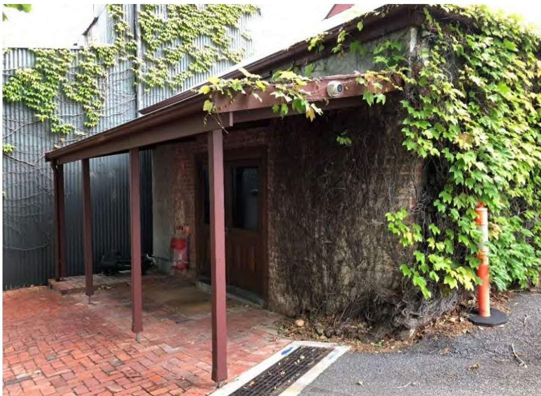
Figure 16: Haselgrove Room exterior (GGA, February 2021)
