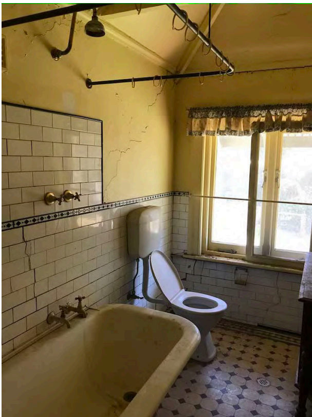
Figure 23: Cracking of masonry and floors of double-storey wing Source: Hosking Willis, 2020
