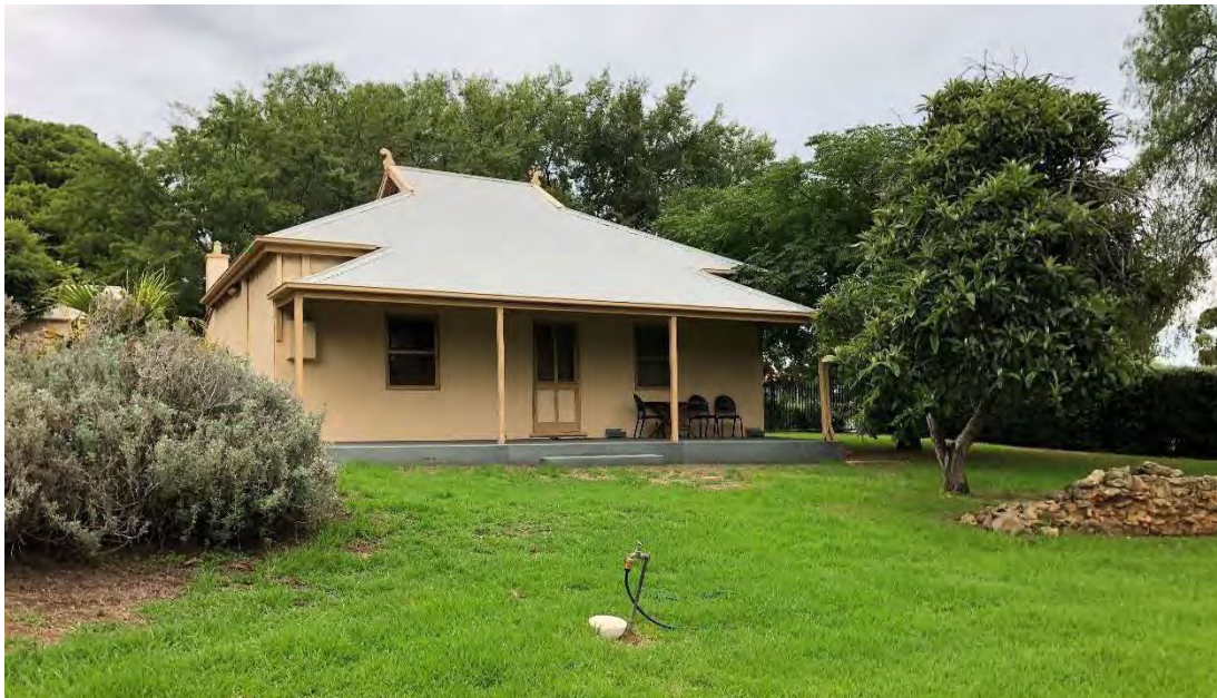
Figure 9: Dwelling, adjacent (but not fronting) Reynell Road, Reynella (GGA, February 2021)
