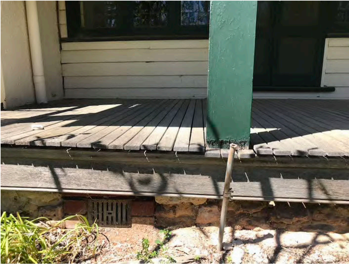
Figure 24: Subfloor masonry walling to verandah of single-storey wing Source: Hosking Willis, 2020
