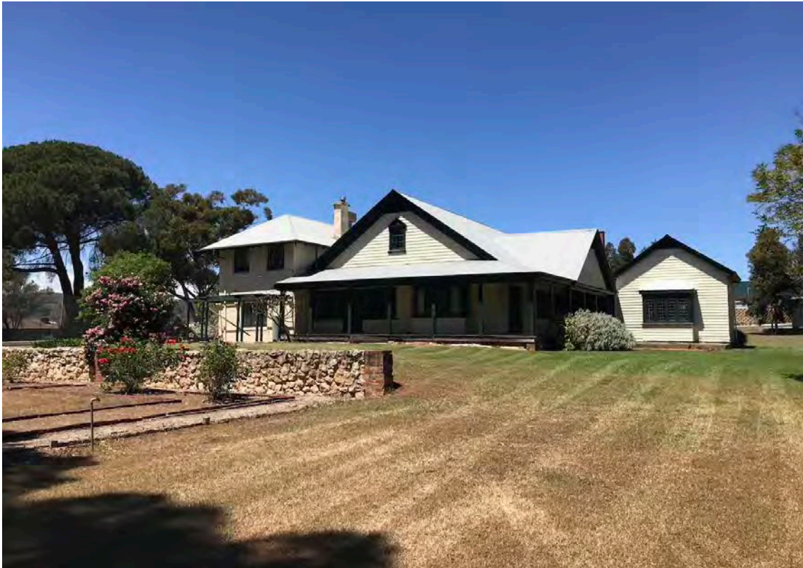
Figure 7: View of Carew Cottage from north west with original timber dwelling (centre) and 'school room' (right)
