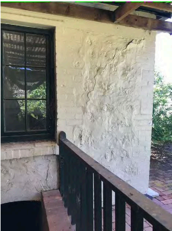
Figure 17: Cracking to masonry walls and interior of (former) kitchen wing
