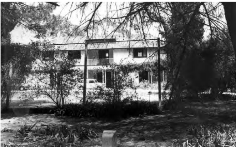
Figure 6: 'Carew Cottage' viewed from Panalatinga Road, 1984 Source: City of Onkaparinga Library, Item 584
