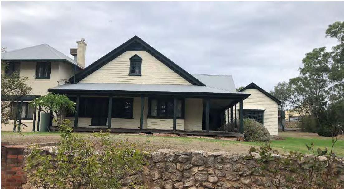
Figure 3: Carew Cottage, off Panalatinga Road, Reynella – viewed from north (GGA, February 2021)
