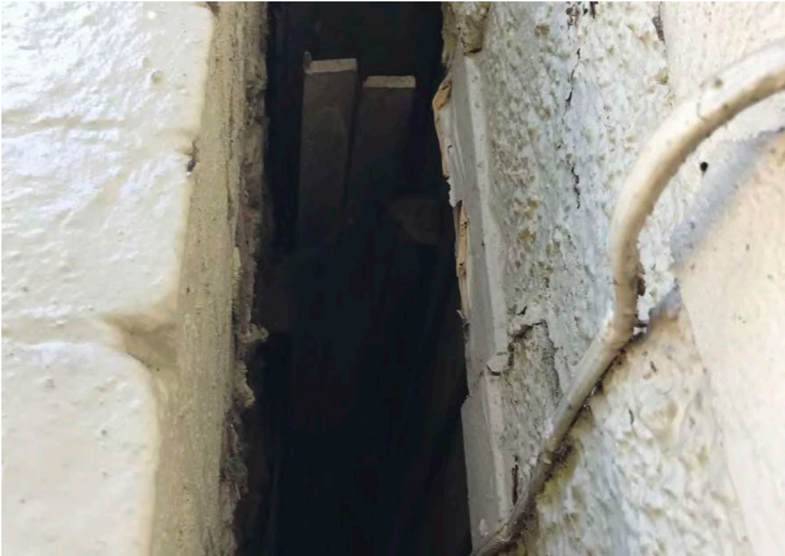
Figure 13: South elevation, junction of timber building and detached stone kitchen wing indicating unfinished north elevation of kitchen
