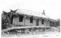
Cottage 31 has original flat iron roofing
