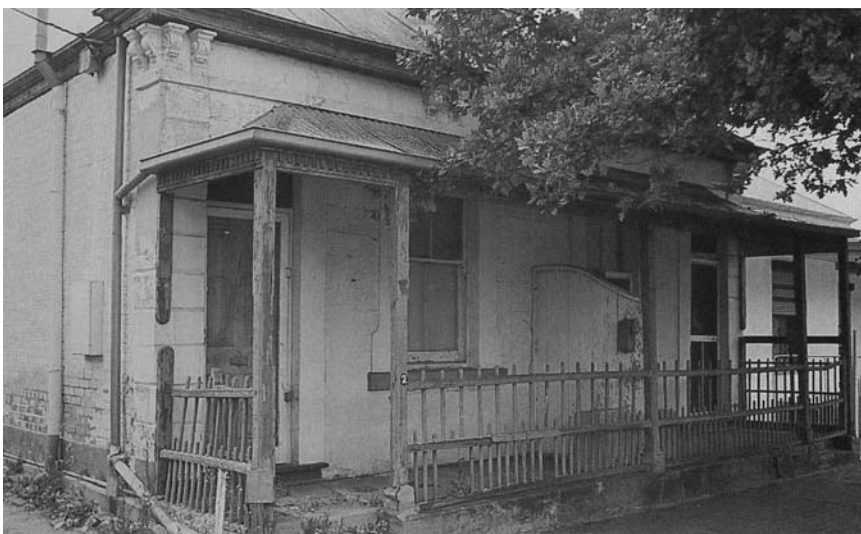
Examples of existing simple timber picket and dowel fences constructed as railing to the narrow verandahs of small 1870s and 1880s single fronted cottages in the city and inner suburbs.
