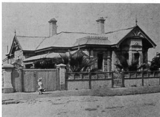
Corrugated iron and timber was used in combination for this fence in Adelaide at the beginning of this century. Note the large vehicle gates repeating the use of corrugated iron.
