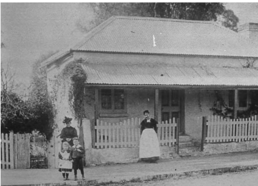
A small cottage in Norwood with its original split paling timber fence in the 1860s, and a new machine-sawn round headed picket fence in 1885. (Kensington and Norwood Council Historic Photo Collection)
