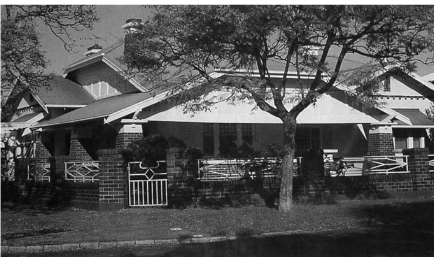
Many 1940s Bungalows had fences constructed in the same materials as the house itself, often utilising wrought iron as an extra decorative element.
