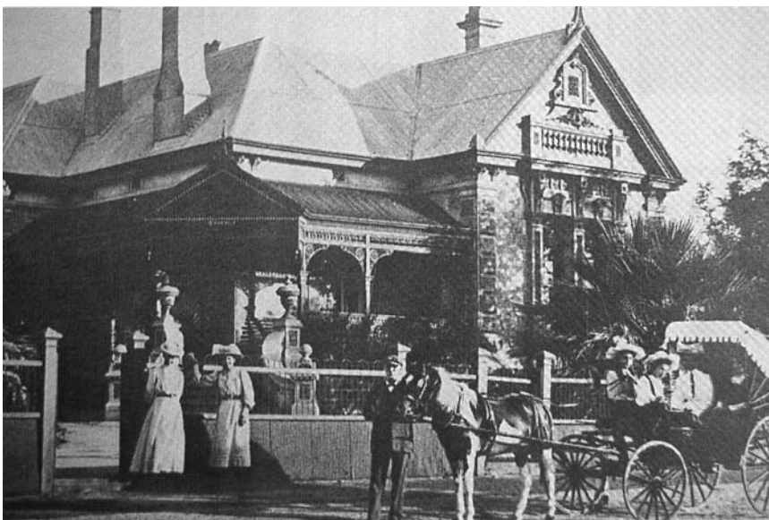
In about 1890, this large St Peters residence had a fence of timber and "ripple iron" (finely fluted corrugated iron) with a top section of woven wire fabric. This is an early example of woven wire. (St Peters Council Historic Photo Collection).
