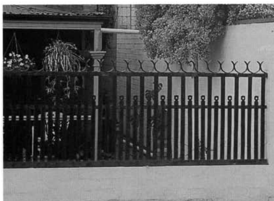
An example of Hume rolled steel fence panels in a picket design, re-used in a new fence to an early cottage.
