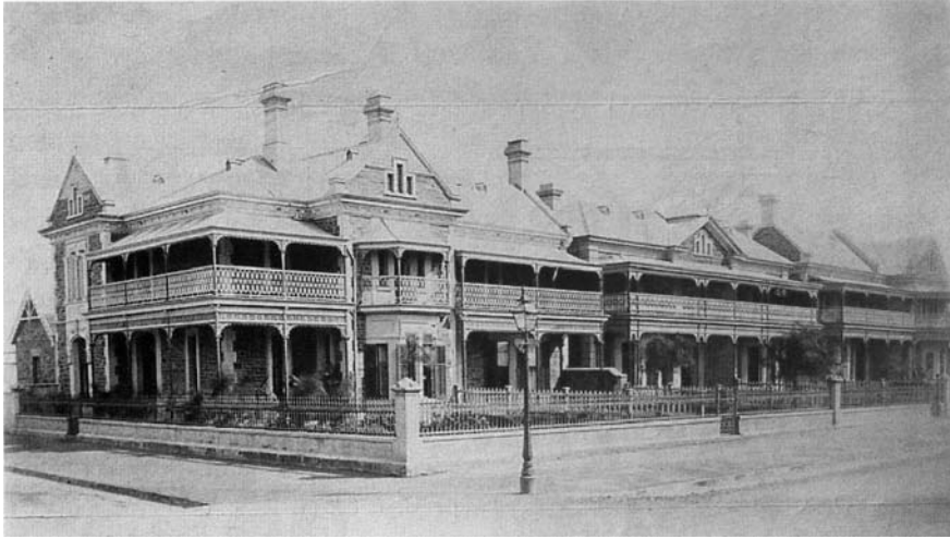
Cast iron and masonry fences at 61-63 Le Fevre Terrace, North Adelaide in the 1880s. These fences are typical for residences of this scale and type. (SSL:M: B6379)
