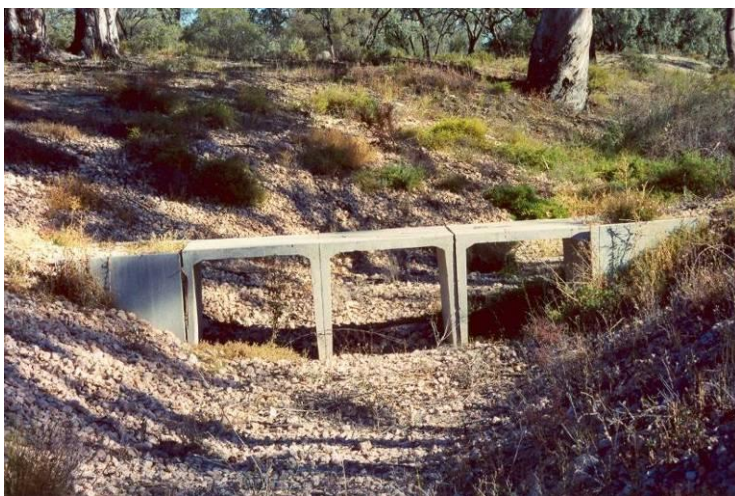
Figure 6: Richard's Creek box culvert
