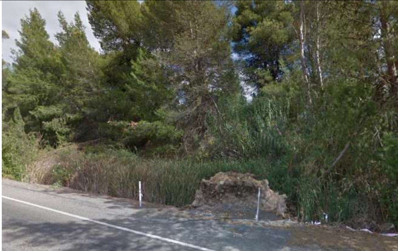
Photo 3. Looking south west from approx. MM 206.05, GPS 287252/6227266. The reeds occur in the deeper part of the creek which is fringed by exotic species including declared weeds. Drainage infrastructure is to be cleaned out, headwalls replaced, and scour protection provided.
