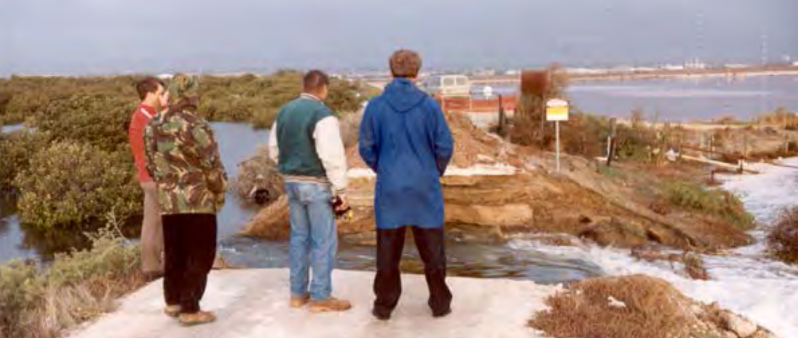
Levee breach, Gillman 1994
