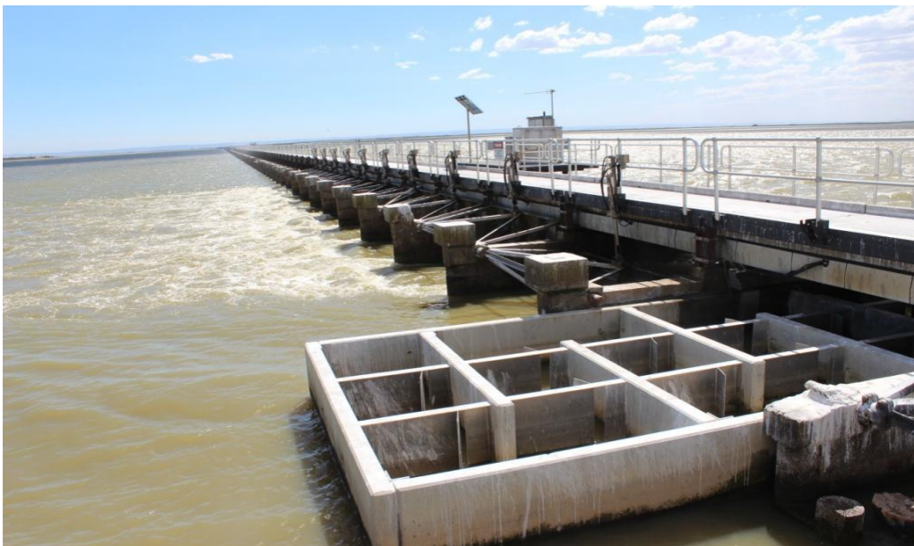
Figure 11 - Small vertical slot fishway in operation at Tauwitschere Barrage
