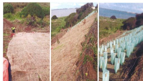
Laying the jute netting after the clearance work at Noonameena and the planting commenced
