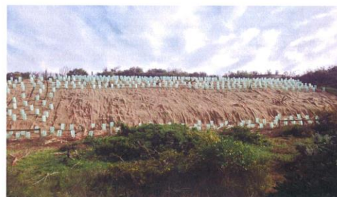
Laying the jute netting after the clearance work at Noonameena and the planting commenced
