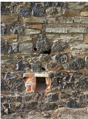
Wall construction - note slag blocks,
