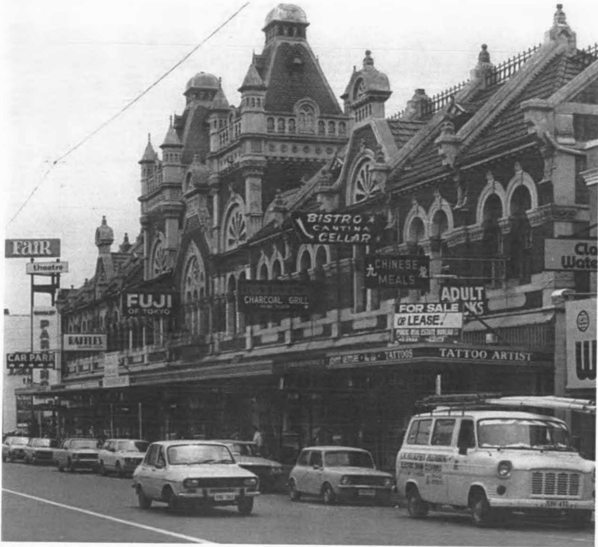
The signage does not respect the building's character and architectural features Hindley St. Adelaide (ACCHS)
