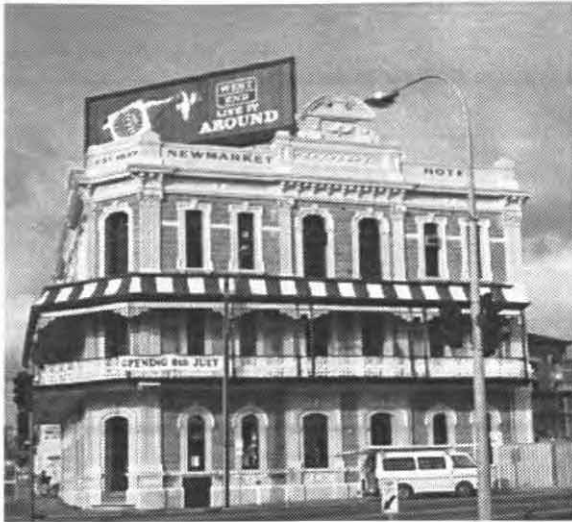
Sky signs, such as this, are very obtrusive and detract from the character of the building.
