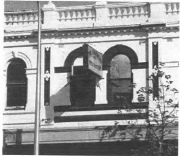
The window in the middle is completely hidden by this large sign. The box sign below looks "stuck" onto the building.
