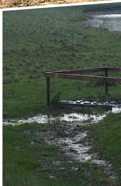
Device inlet with wing walls on each side to direct flows into the inlet.
