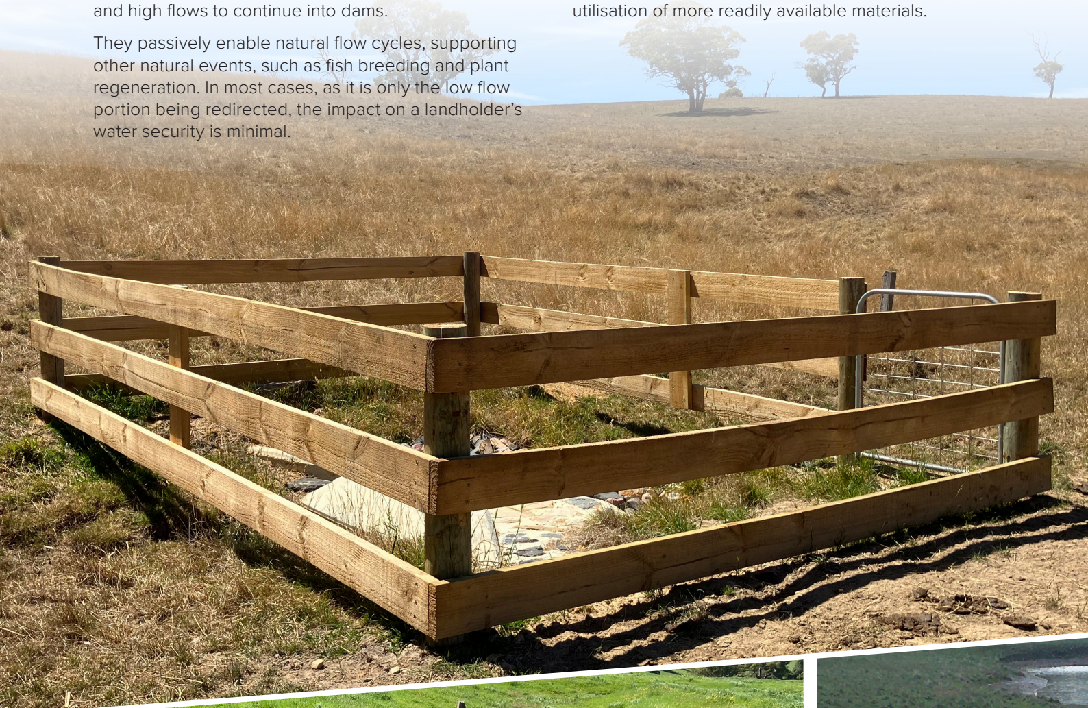
Device inlet with wing walls on each side to direct flows into the inlet.
