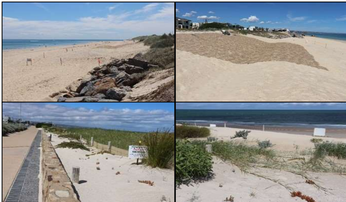
Figure 20: Dune condition on the replenished incipient dune and foredune stoss with jute mesh covering (top) and landward slope (bottom).
