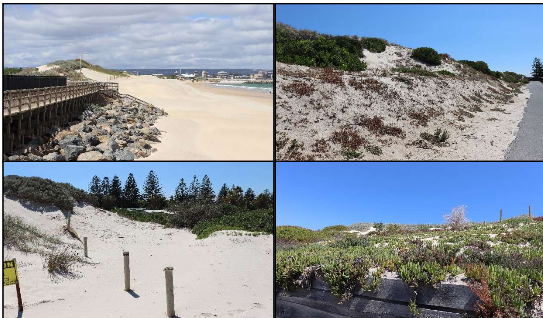
Figure 41: Sand replenishment building volume on the stoss slope (top left) and condition of the landward slope showing mostly good vegetation cover, with some bare patches and a moderate to high level of weeds (other).
