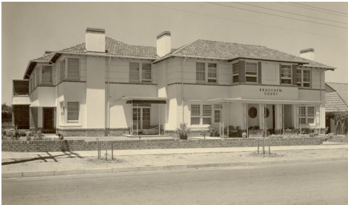
Image: Bruceden Court (flats), c.1941, showing front elevation of duplex (two-storey) flats
