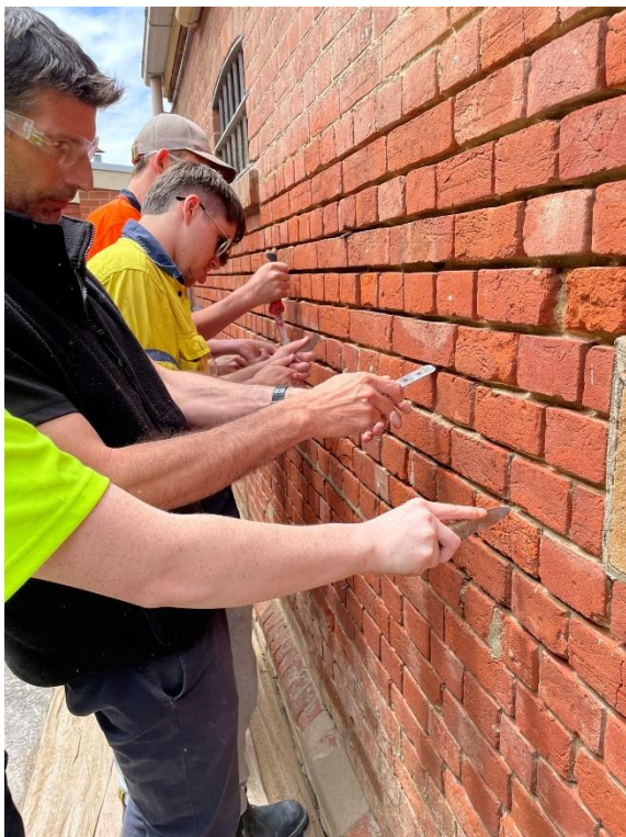
Image 1: Removing previous concrete. Image 2: Repointing with lime mortar.
