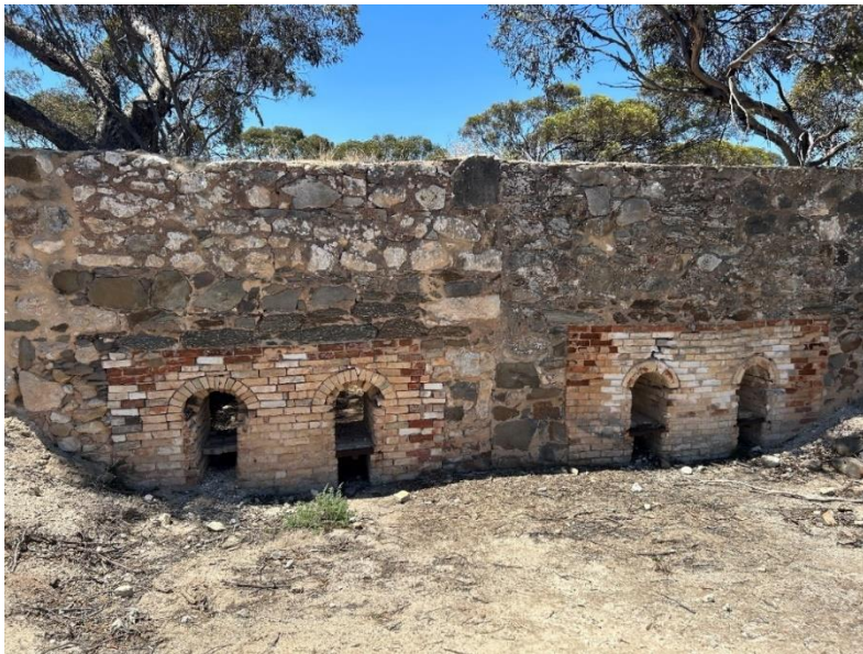
Image: The D-type lime kilns built by George Green in the late nineteenth century.
