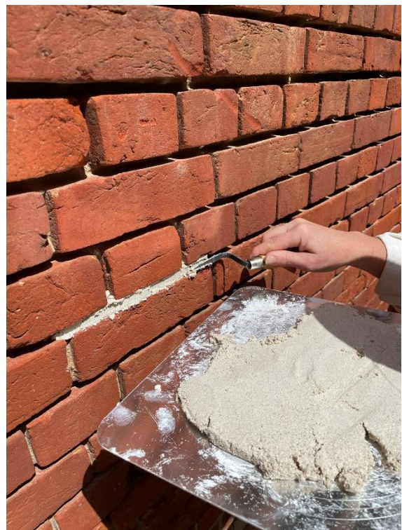
Image 1: Removing previous concrete. Image 2: Repointing with lime mortar.
