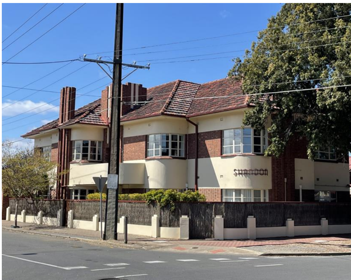
Image: Shandon (flats), 88 Moseley Street, Glenelg South Source: DEW Files, 27 September 2023
