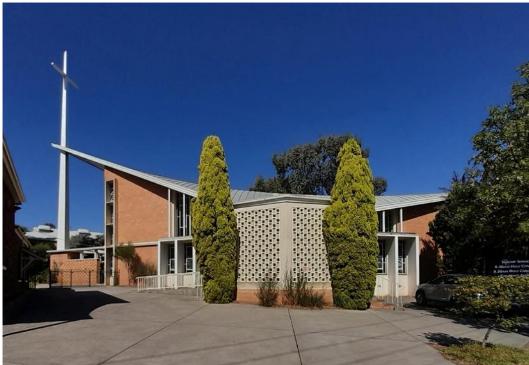
Image: St David's Anglican Church. Source: DEW files.
