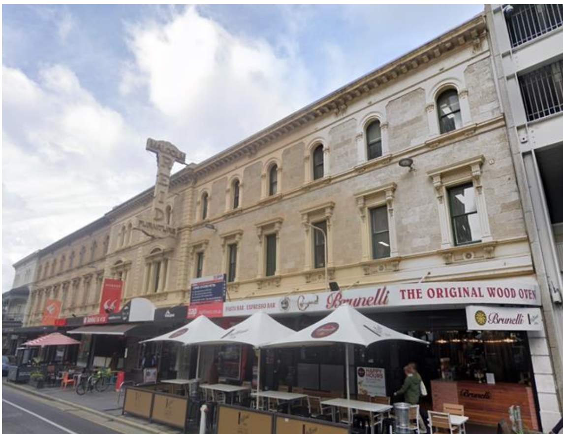
187-195 Rundle Street, August 2023. Source: Google Maps
