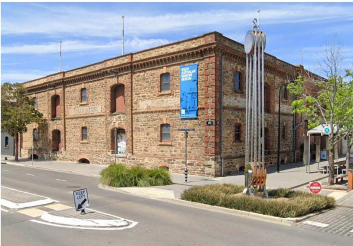
Former Elder's Bond and Free Stores, showing Divett and Lipson Street elevations of 1856-1857 store after conversion to South Australian Maritime Museum display and interpretive centre, 2021.
