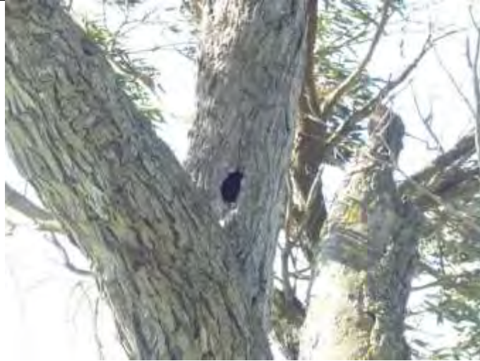
Figure 47. One small hollow observed in Tree 22.
