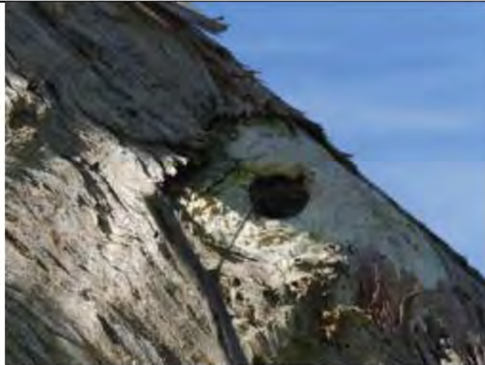
Figure 24. One small hollow observed in Tree 11.
