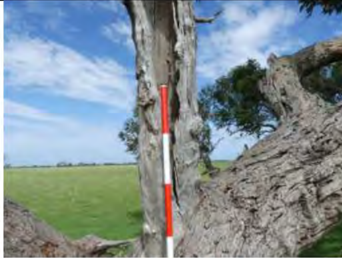
Figure 8. One large hollow observed in Tree 2.
