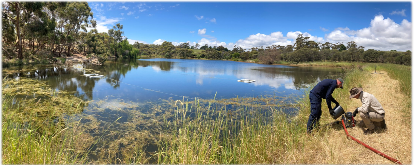
Above, Murray and Damian trial flows at Glenthorne National Park. Siphons are used to lower the dam water level to enable works around the embankment. This may be more suitable to dams where trenching is a challenge. Watch this space!
