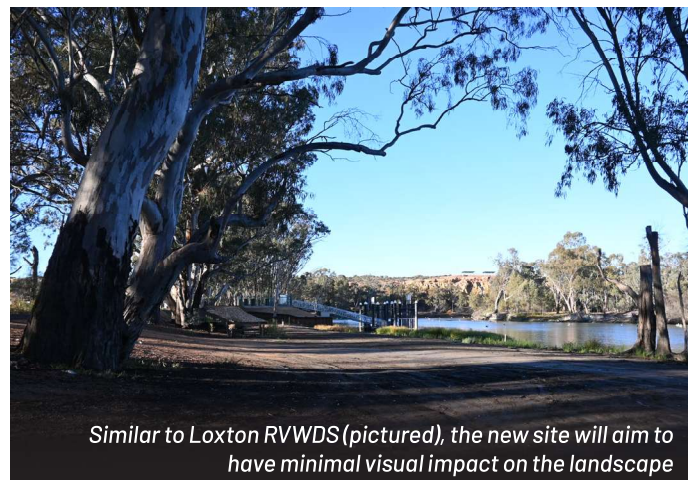
The new station will be similar in appearance to the Loxton RVWDS
