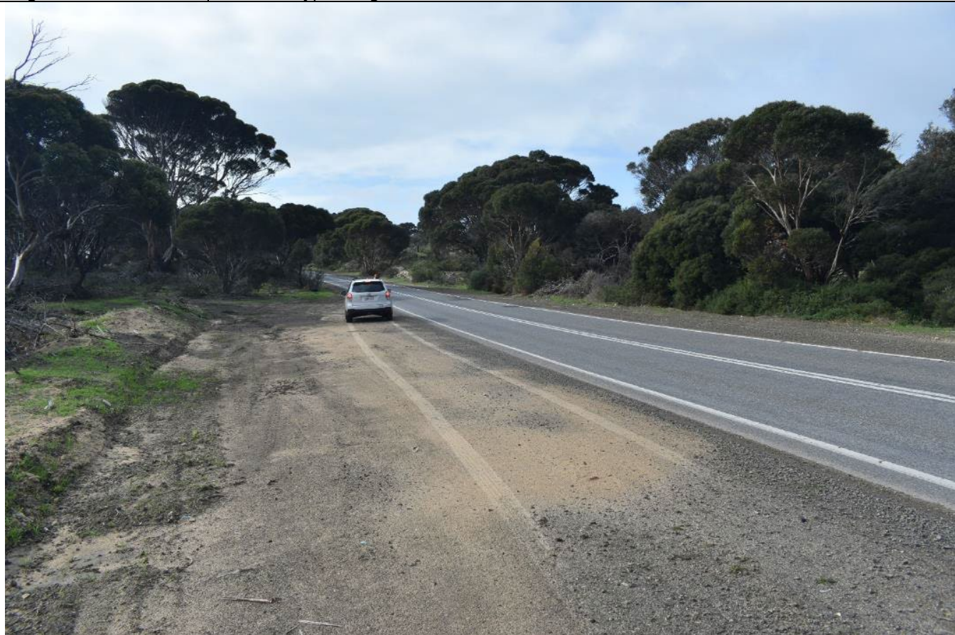
Photo 3. Facing northeast, MM43.1 LHS (works begin ahead of the vehicle)
