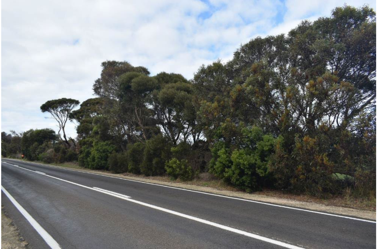
Photo 1. Facing south, MM 23.7 RHS
