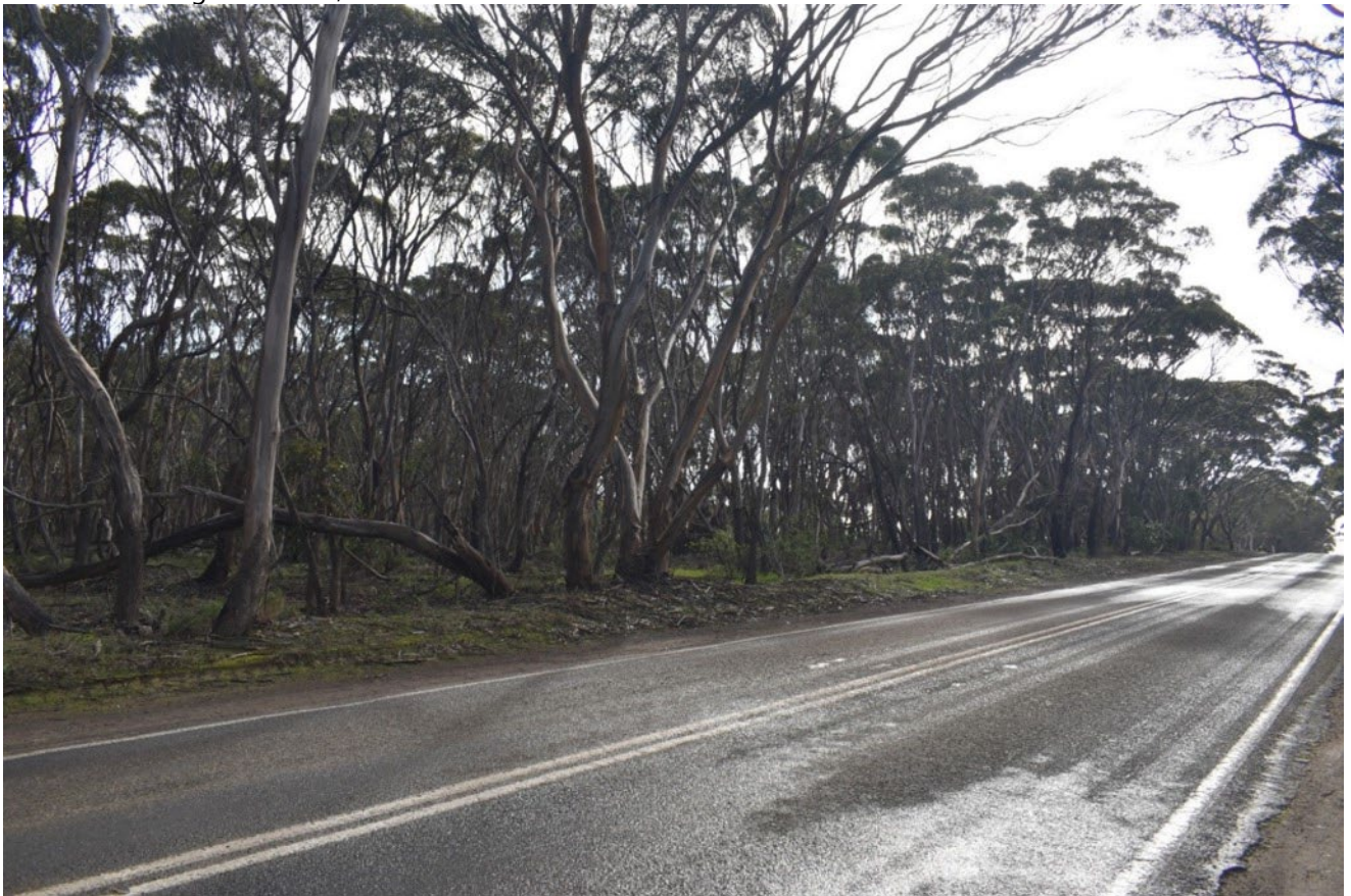
Photo 7. Facing north, MM 49.6 LHS
