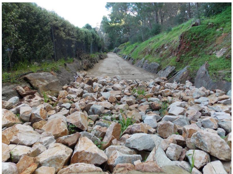
Repaired stormwater overflow Conifer Place
