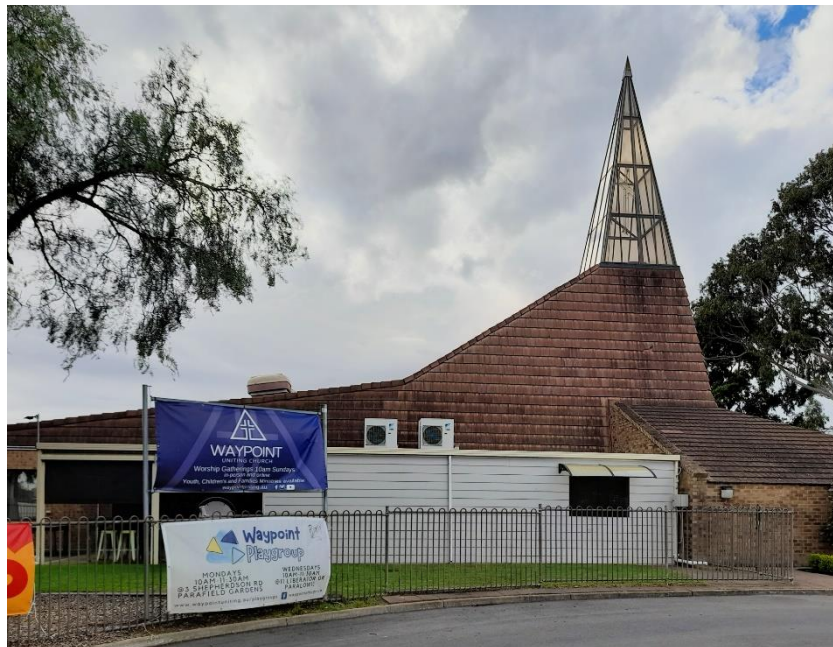
Former Parafield Gardens Uniting Church, note long tiled roof extension on left (gently sloping section) c.2001 and enclosed pergola addition c.2010 and c.2021
