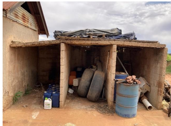
Concrete brick addition to cell block.
