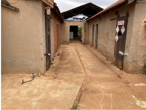
Cell Block showing the cells facing the central corridor, note the drain and sliding door.
