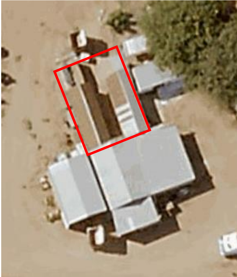
Camp 10 Detention Cell Block, Meru Country, Yeo Road, Loveday CT 5958/949 A8 D 69443 Hundred of Loveday
