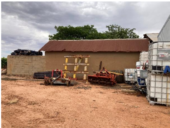
Exterior wall of the cell block.
