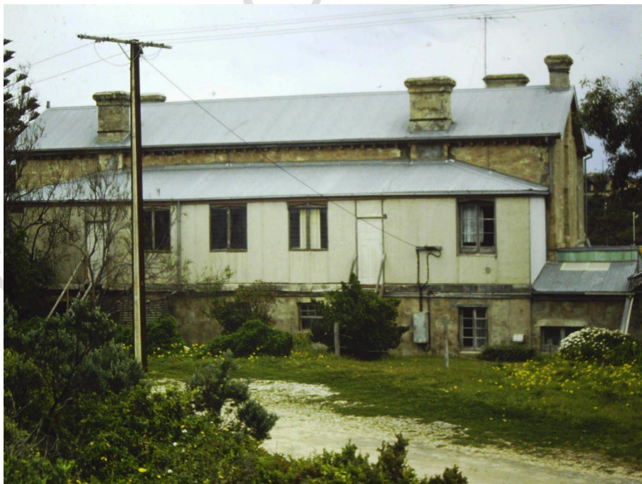
Northern elevation of Karatta House, c.1983.
