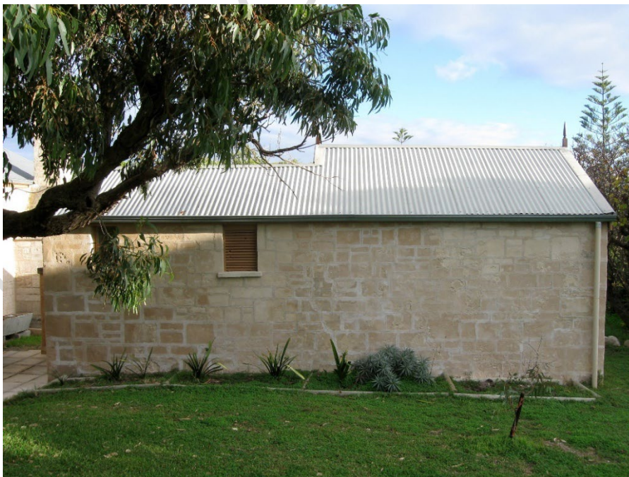
Northern elevation of harness room, woodshed and water closet outbuilding after repointing, c.2010.
