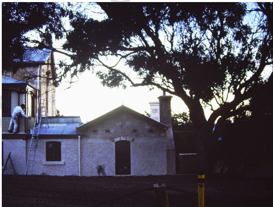
The servants' quarters after conservation work and repointing, c.1990.
