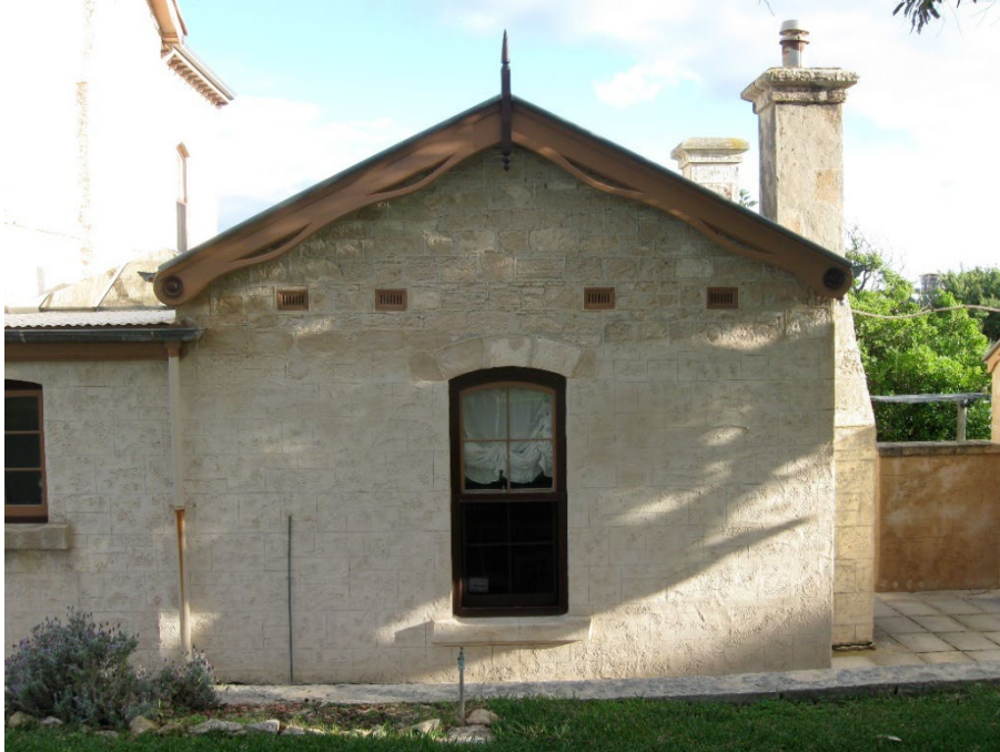
Servants' Quarters after repointing, c.2010.
