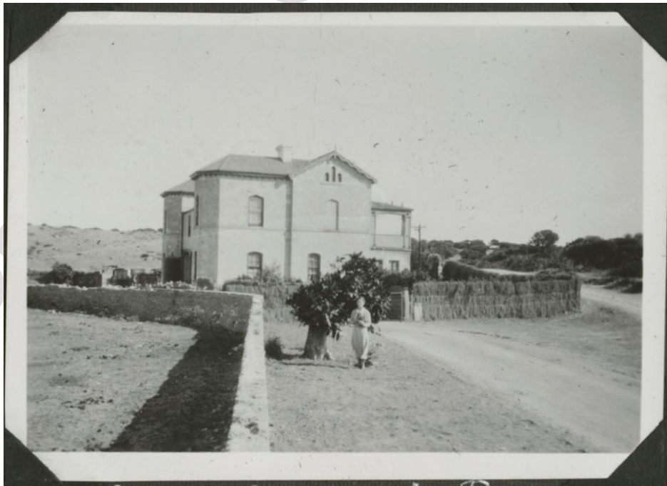
Eastern elevation of Karatta House showing two front wings, c.1936.
