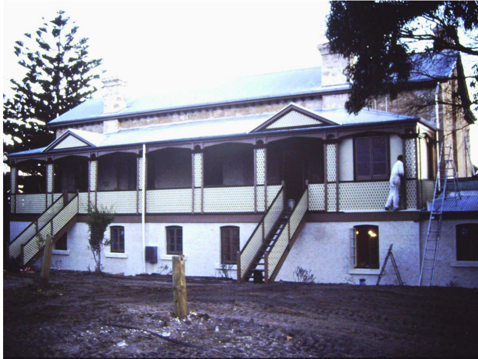
Northern verandah being renovated, c.1990.
