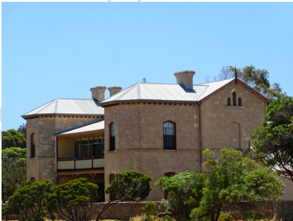
Eastern elevation of Karatta House, 2016.
