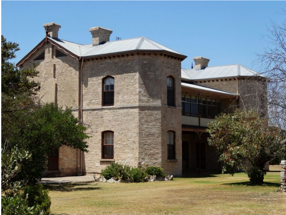
Western elevation of Karatta House, 2016.
