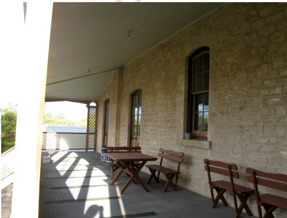
Front verandah showing repointing, c.2010.
