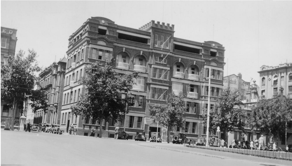
The 5 th floor extension of Gawler Chambers under construction, 1935.
