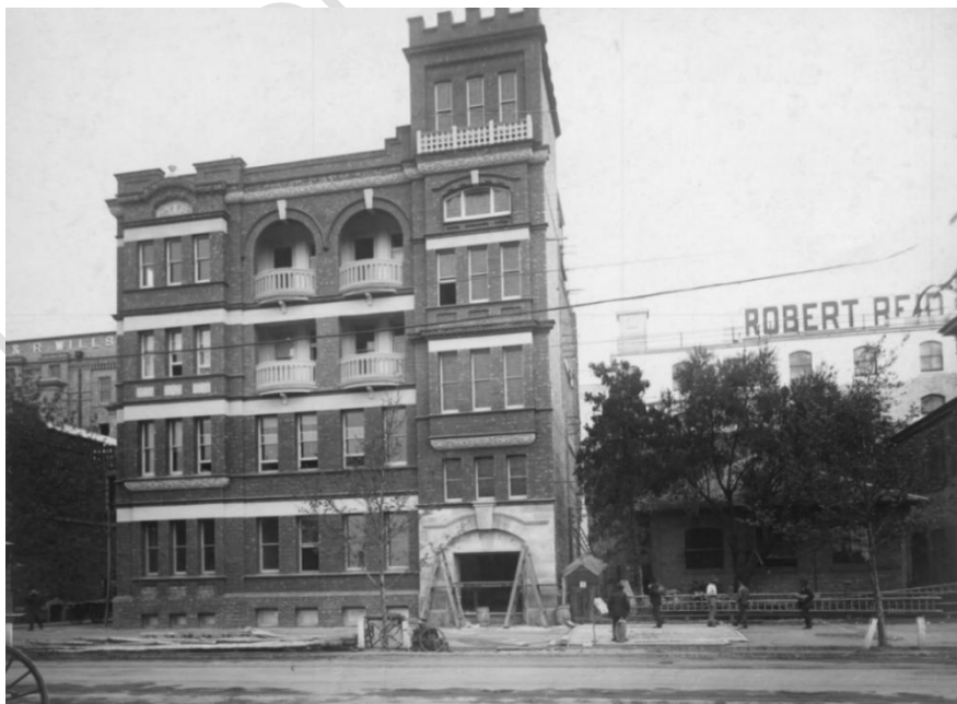
Eastern side of Gawler Chambers prior to erection of western side, c.1913.
