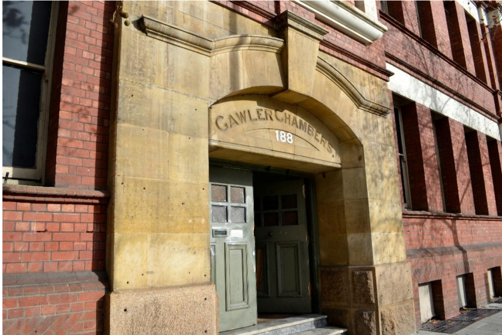
Main entrance on northern elevation, 2014.
