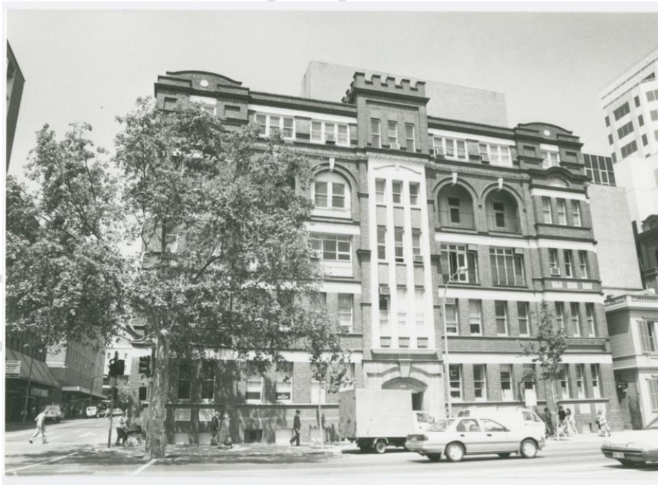
Gawler Chambers, c.1991. Note the 5 th floor addition, rendered concrete fluting added to the tower and removal of balconies. All alterations occurred between the 1930s and 1960s.
