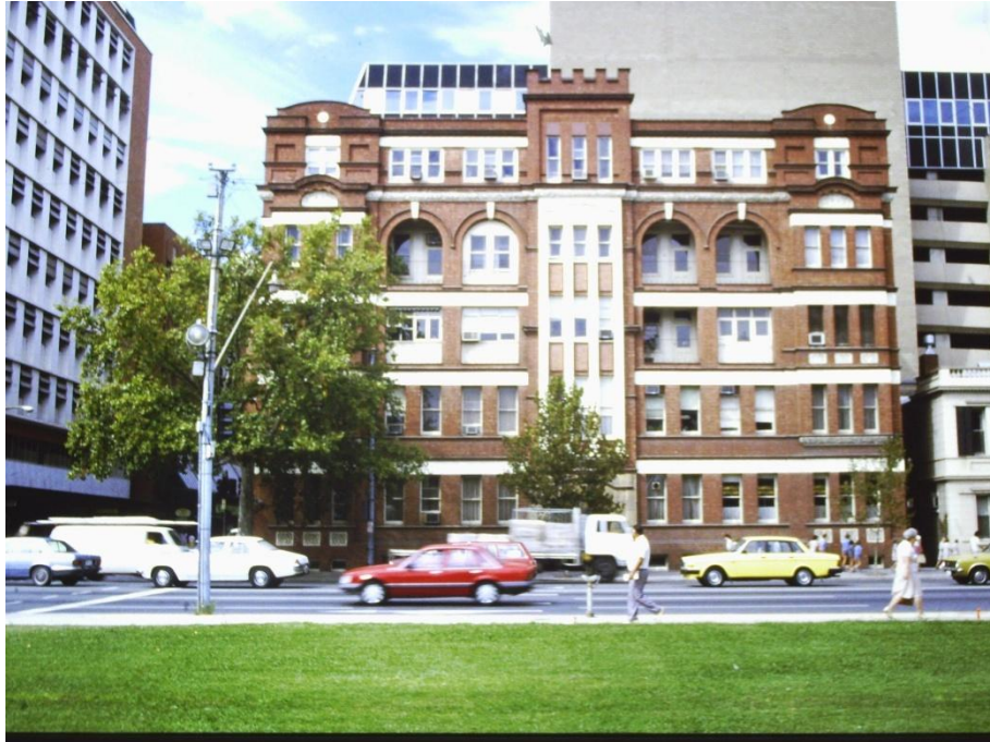
Northern elevation of Gawler Chambers, c.1990s.
