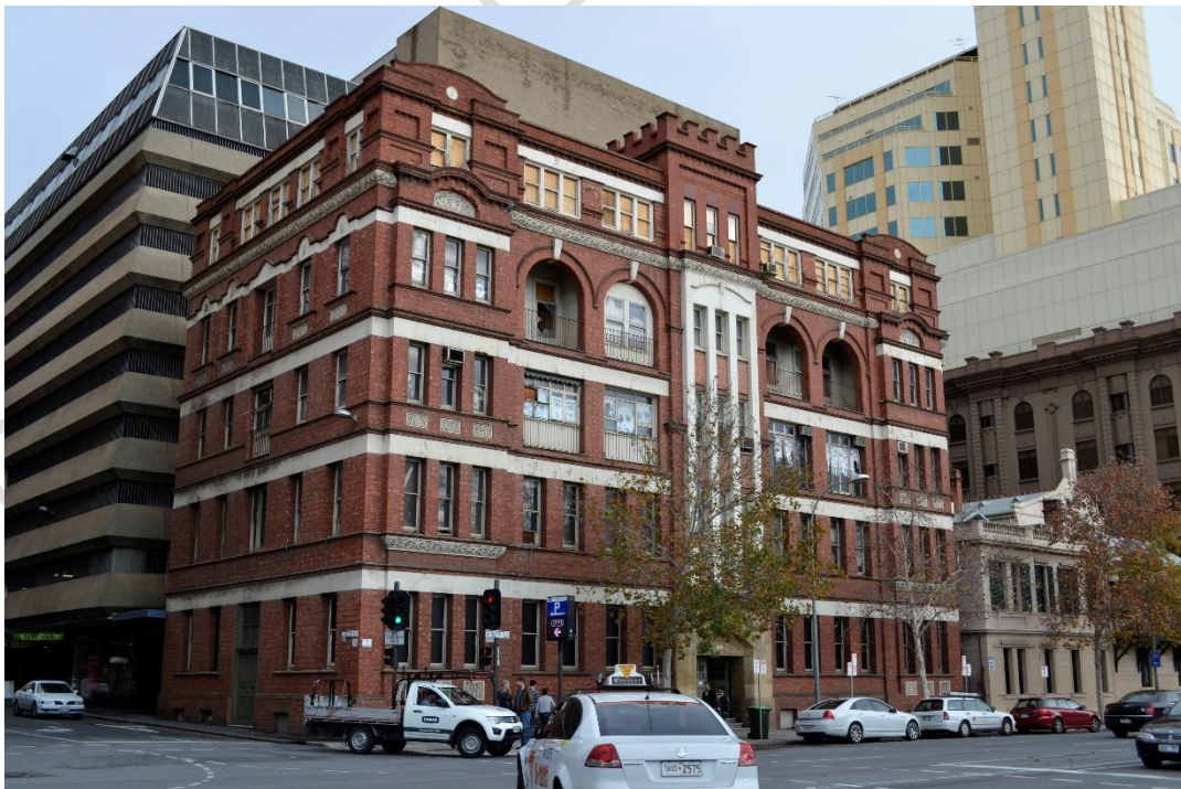
Condition of exterior, 2014.
