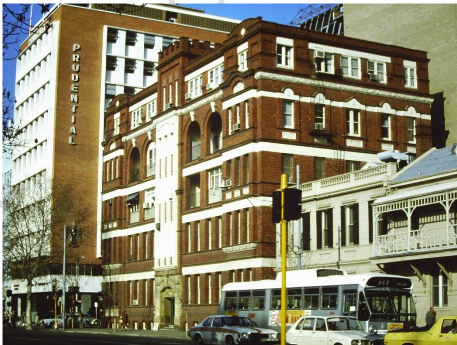
North-west corner of Gawler Chambers, c.1990s.
