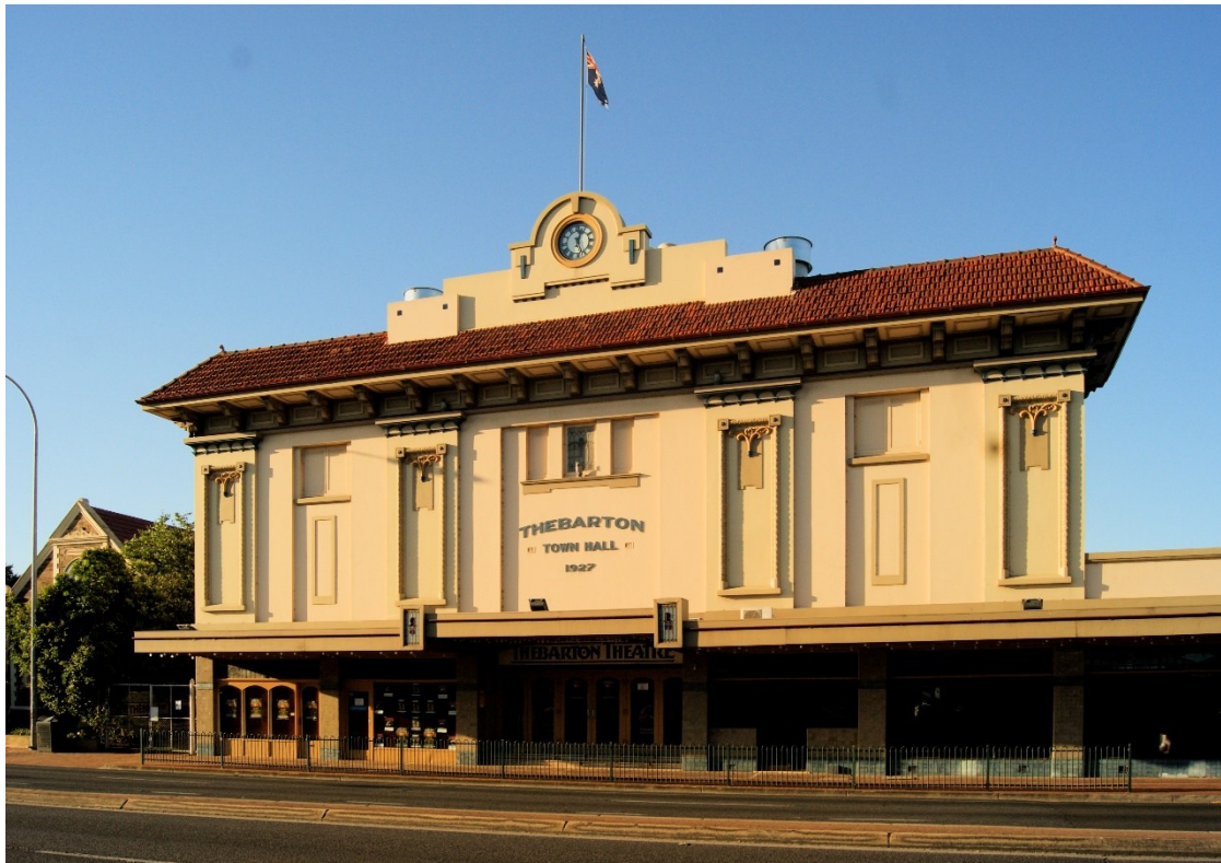
Former Thebarton Town Hall Complex SHP 10645, 2 January 2022.
