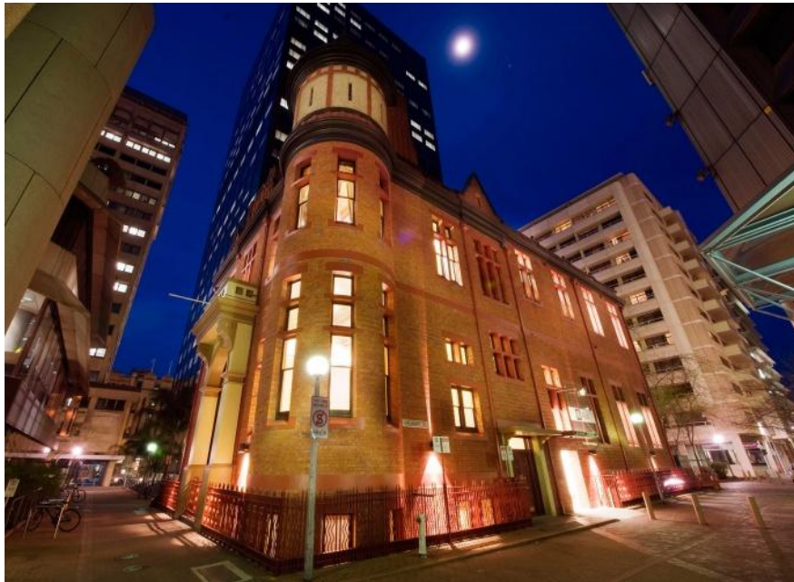
The Former Stock Exchange of Adelaide following completion of renovations in 2007.
