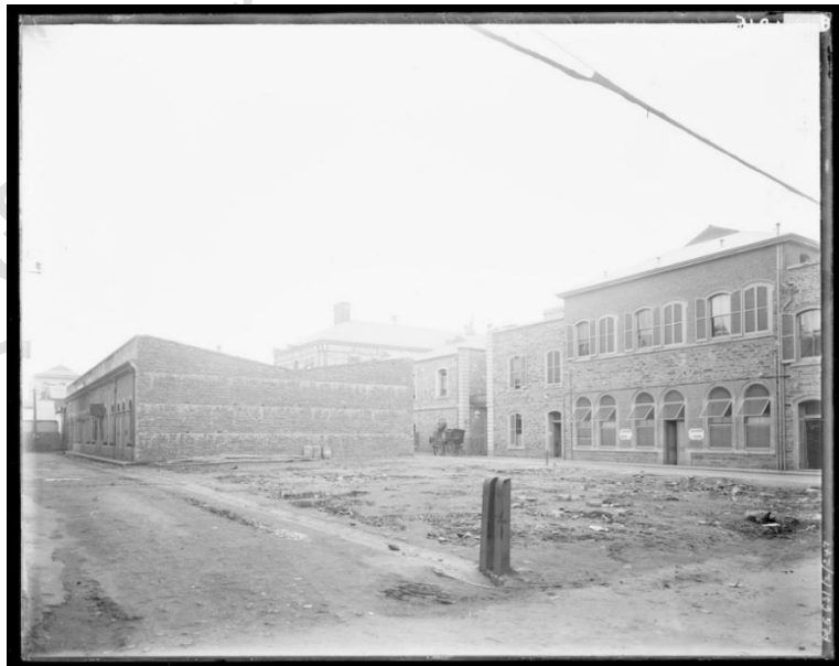
The site of the new Stock Exchange of Adelaide building on Exchange Place and McHenry Street, Adelaide c.1900.
