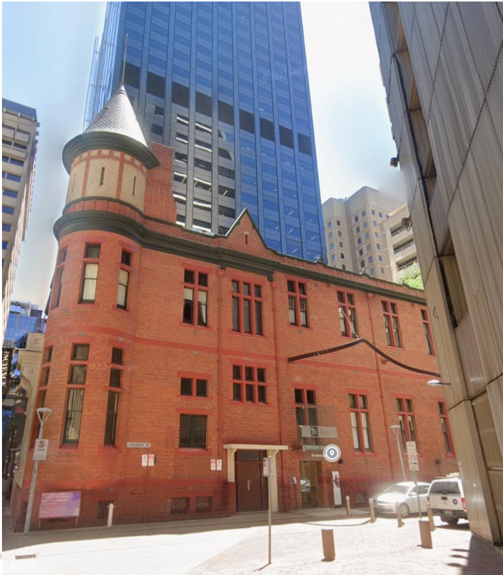
Former Stock Exchange of Adelaide SHP 11580, c. 2020.
