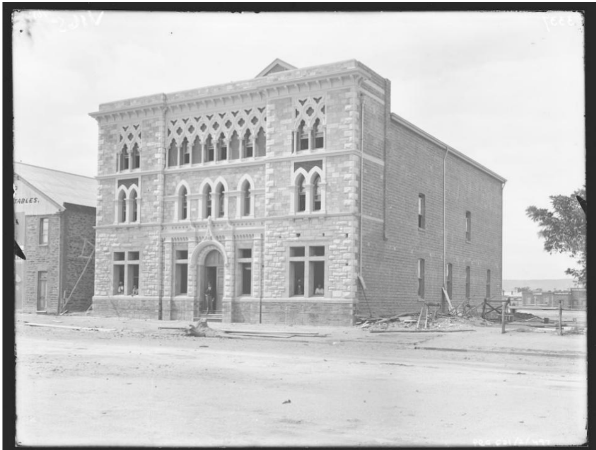
Former Our Boys' Institute Building (Façade) SHP 10890, 1897.
