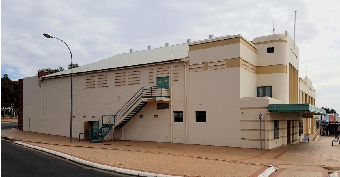
Bonney Theatre Complex, northern side showing escape stairs. Note steel shutters over windows.
