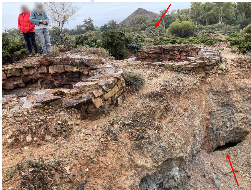
The two lime kilns side by side. Note the partially visible firing port and iron rod (indicated by arrows) on the western kiln to the bottom right of the image.
