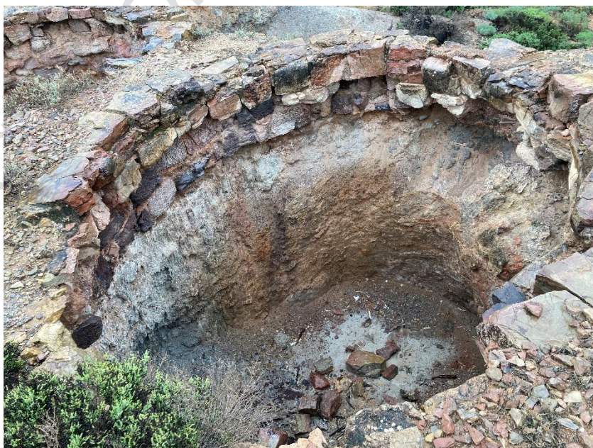
Interior of the eastern kiln, showing dirt and debris filling the shaft. Note the interior is not lined.
