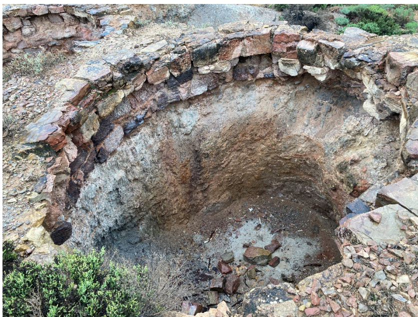
Interior of the eastern kiln, showing dirt and debris filling the shaft. Note the interior is not lined.
