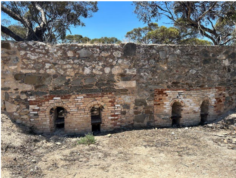
Green Farm Lime Kilns, Monarto (SHP 26598)
