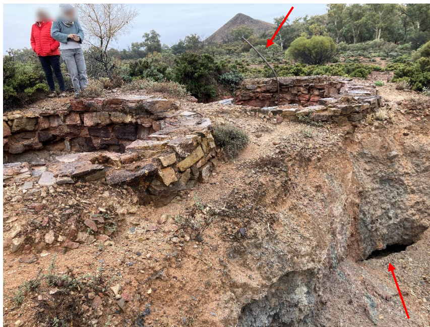
The two lime kilns side by side. Note the partially visible firing port and iron rod (indicated by arrows) on the western kiln to the bottom right of the image.
