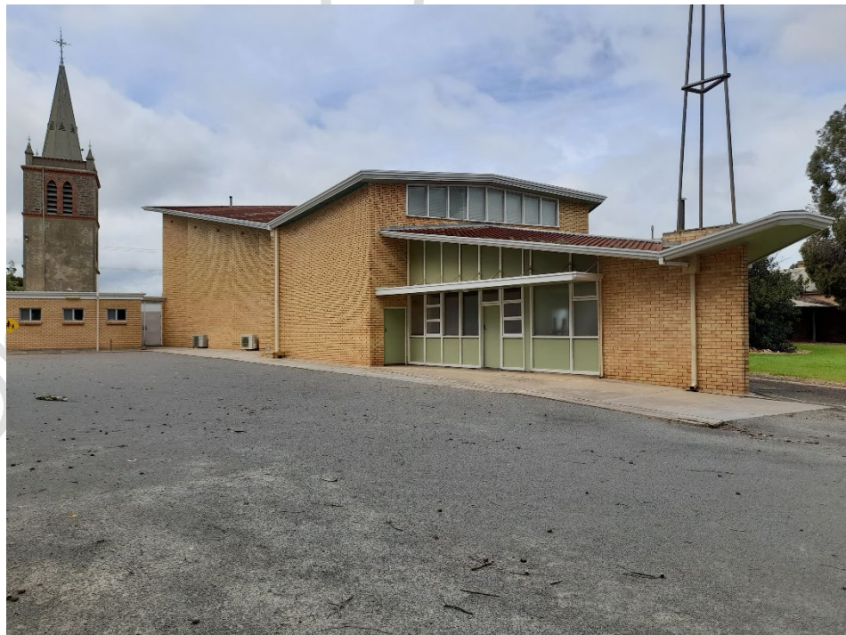
Strait Gate Lutheran Church, northern and western elevations, note butterfly roof form.
