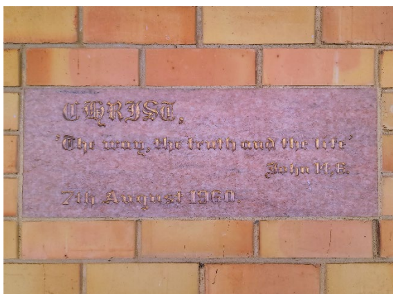
Foundation stone dated 7 August 1960.
