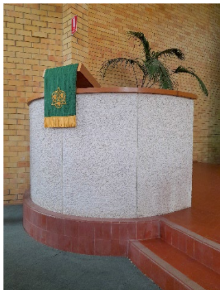
Pulpit in coarse aggregate concrete.
