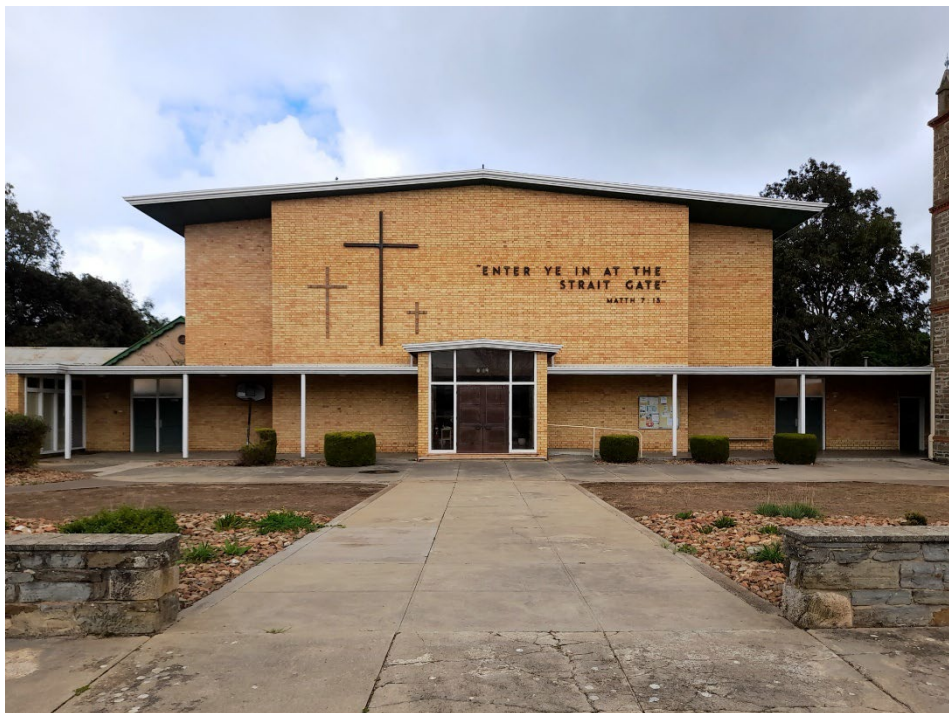
Strait Gate Lutheran Church, exterior, street elevation.
