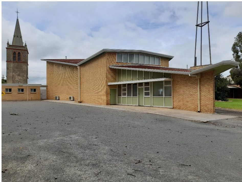
Strait Gate Lutheran Church, northern and western elevations, note butterfly roof form.
