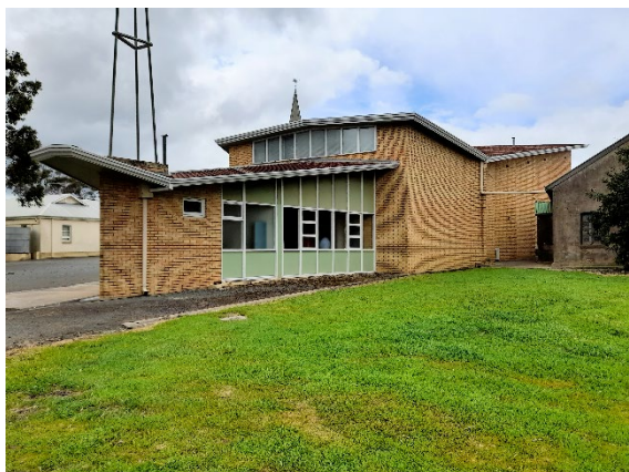
Southern and western elevations.
