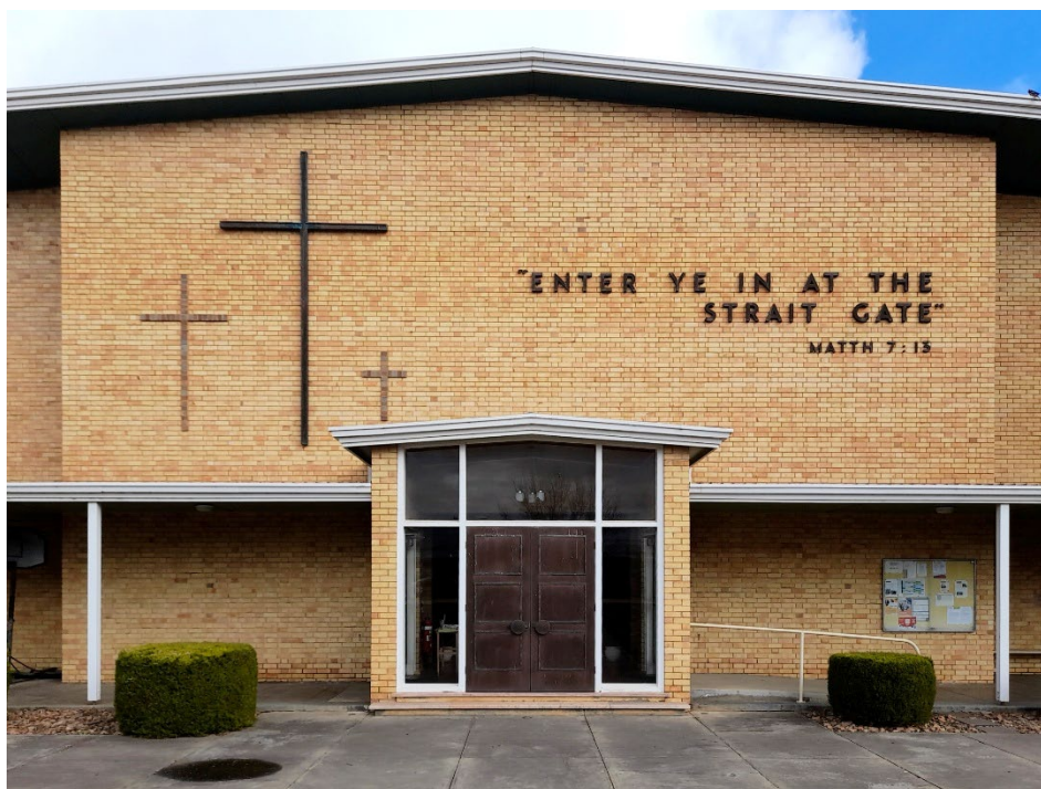
Strait Gate Lutheran Church, exterior, street elevation, note quotation in copper letters.
