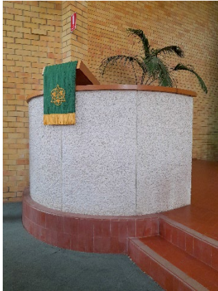
Pulpit in coarse aggregate concrete.
