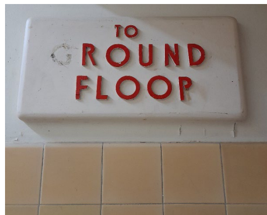
Original tiles and signage in eastern stairwell.
