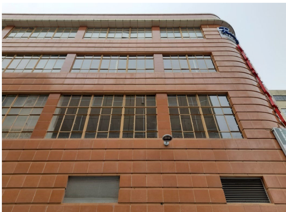
Eastern elevation, note structural columns passing through window openings.
