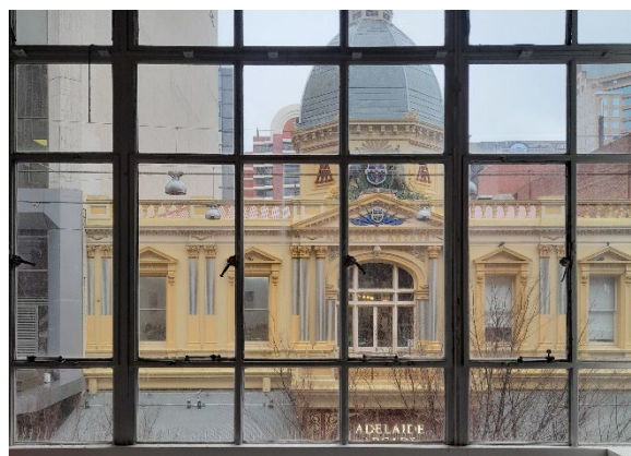
Original non-ferrous metal window frames.
