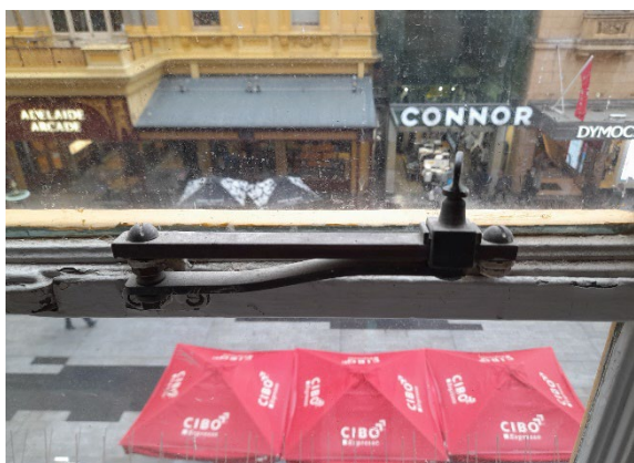
Original window frame hinge hardware.
