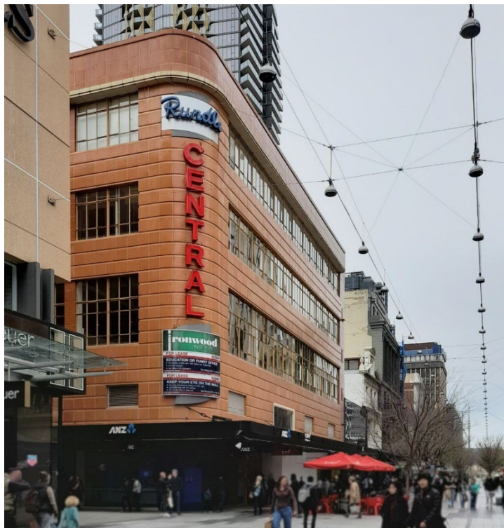
Former G. J. Coles & Company Adelaide Store, southwestern corner.
