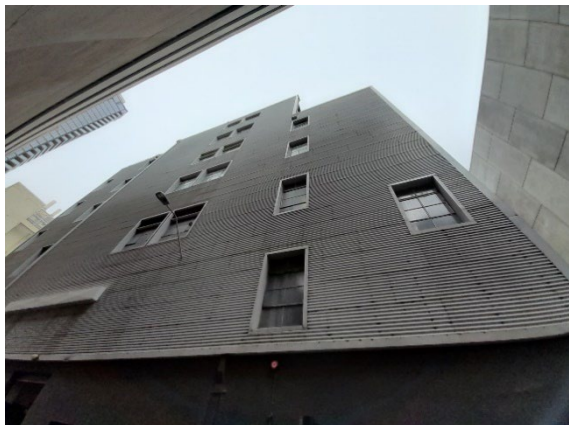
Northern elevation, showing c.2000 cladding.
