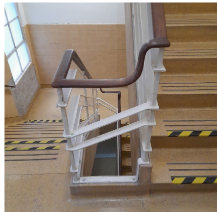
Western stairwell balustrade and terrazzo treads and landing.
