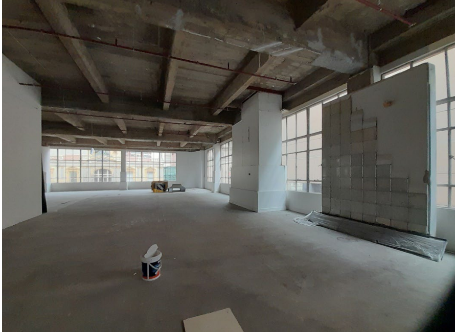
First floor interior (former cafeteria) looking south.
