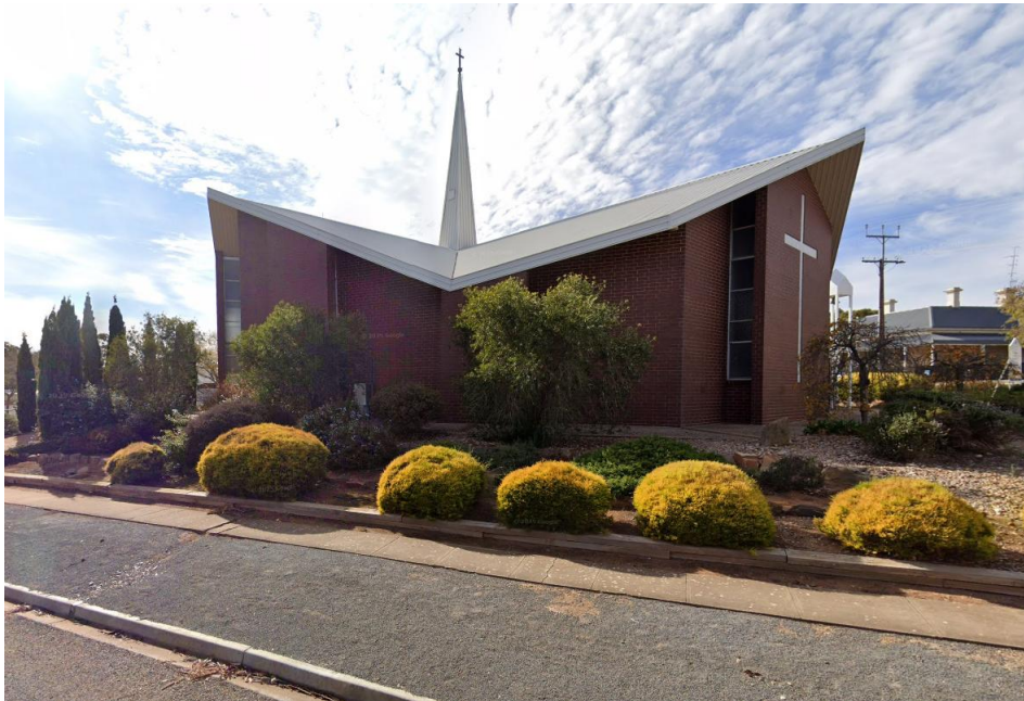
St John's Lutheran Church, southern and western elevations.
