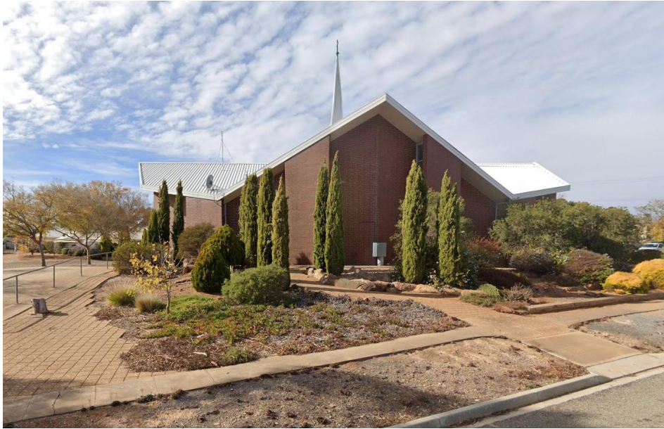
St John's Lutheran Church, western elevation.
