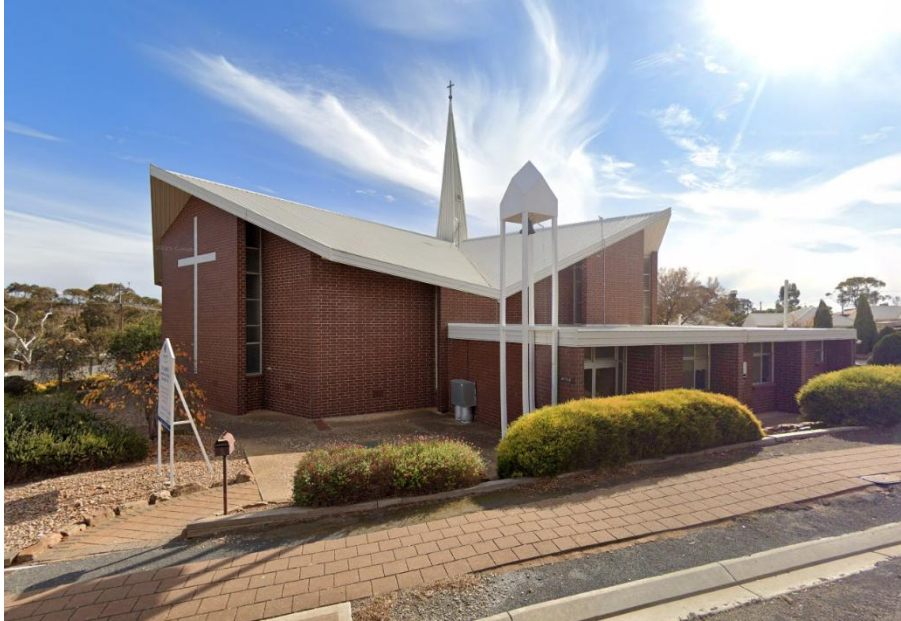
St John's Lutheran Church, southern and eastern elevations, note freestanding belfry and single-storey narthex and administration wing.
