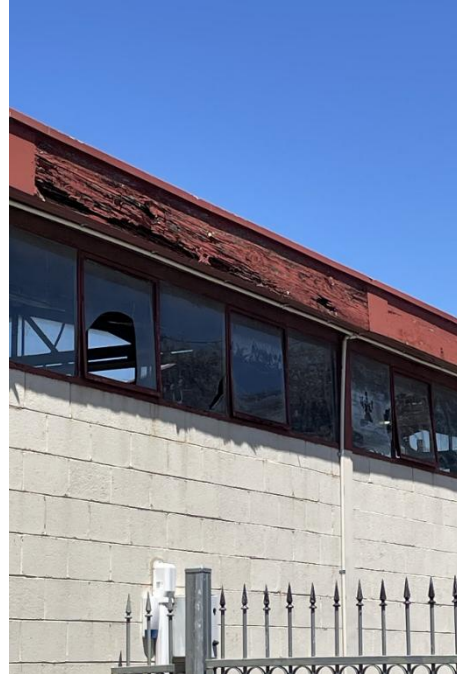
Indicative damage to facias (rot) and glass.
