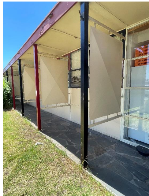
Eave at southern elevation with steel posts and fins.
