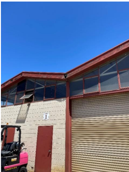
Indicative damage to facias on northern elevation.
