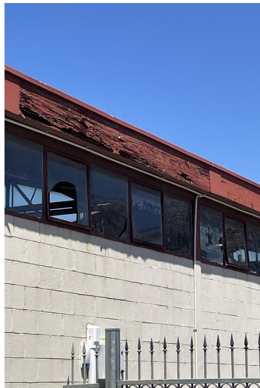
Indicative damage to fascias (rot) and glass.
