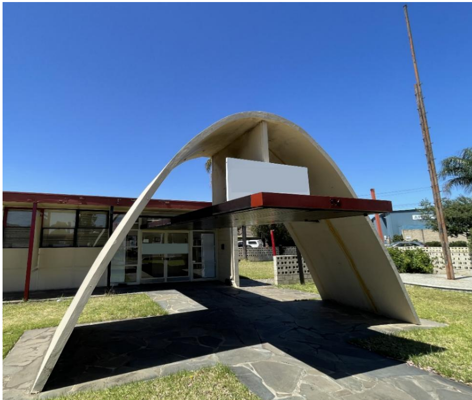
Reinforced concrete parabolic arch supporting canopy fronting the Sisalkraft Factory Complex (business signage obscured).
