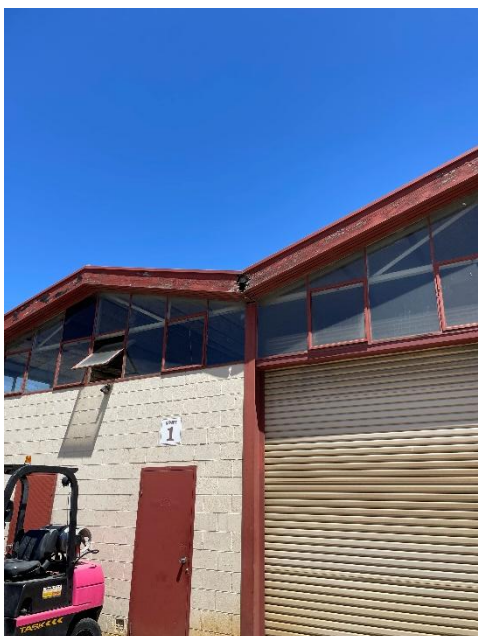
Indicative damage to fascias on northern elevation.
