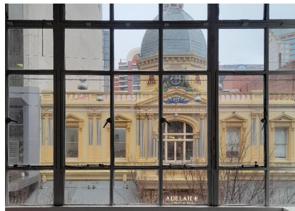
Original non-ferrous metal window frames.
