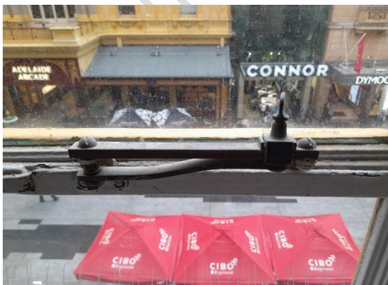
Original window frame hinge hardware.
