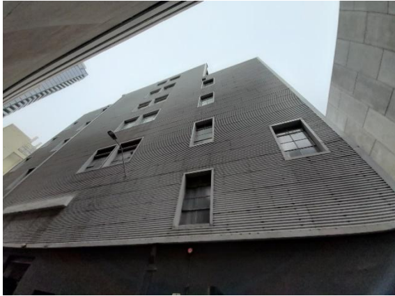
Northern elevation, showing c.2000 cladding.
