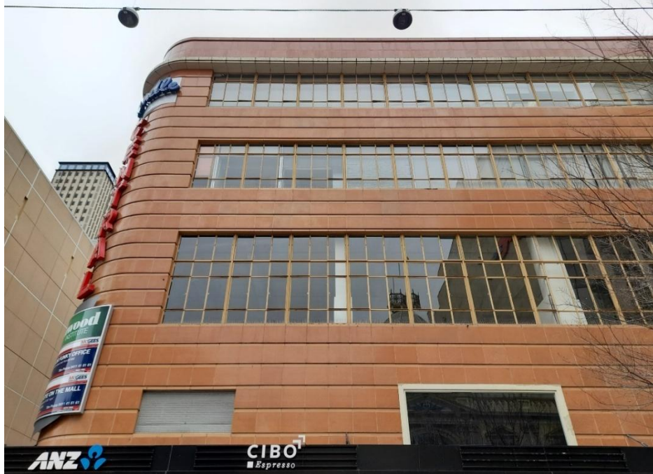
Southern elevation, note wide spans of ribbon window openings with structural columns behind (columns boxed out with non-original fabric).
