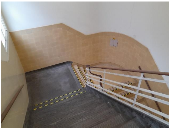
Western stairwell showing transition from concrete treads and landing to terrazzo section to lower floors.
