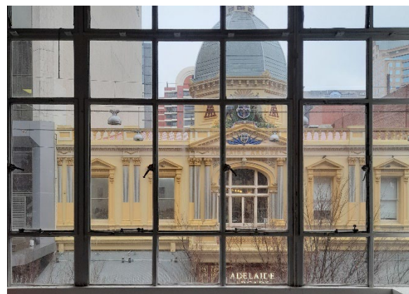
Original non-ferrous metal window frames.
