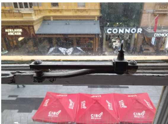
Original window frame hinge hardware.
