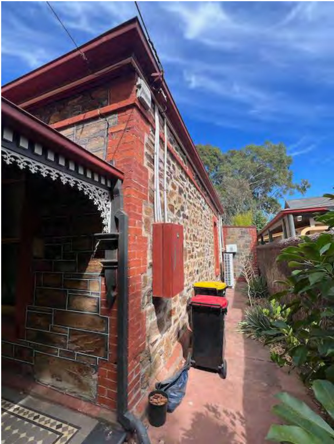
Side wall underpinned, straightened and plumbed for about $20K by 'urathane solutions'
